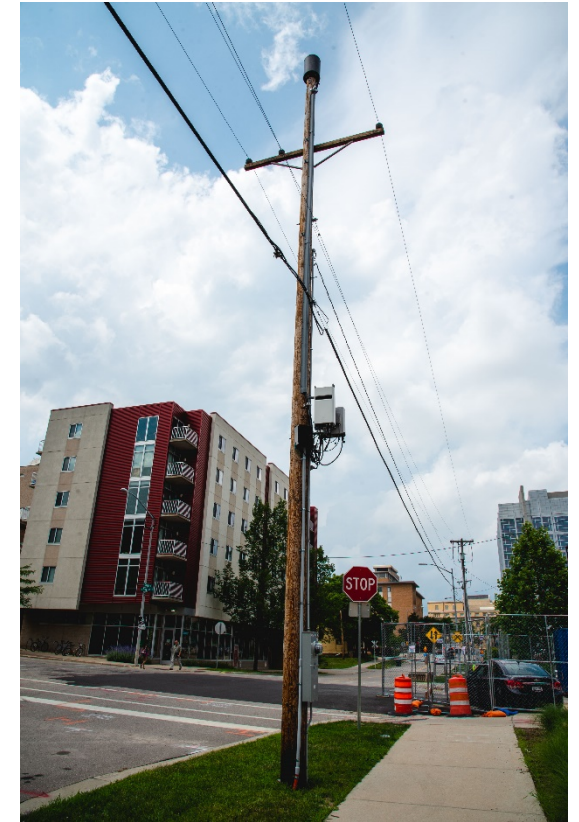
Small cell installation on an MG&E pole on Charter St. & Dayton St.
