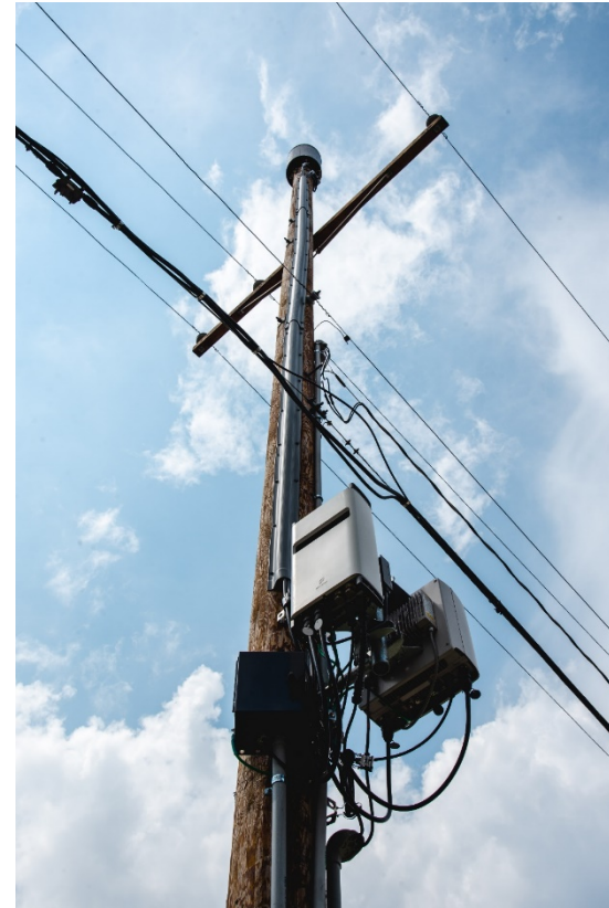
Small cell installation on an MG&E pole on Charter St. & Dayton St.
