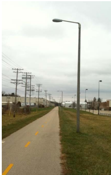
From left to right: Concrete pole on path, same as on residential streets (25 ft); 30 ft with twin side of pole fixtures on John Nolen; Residential Concrete Post Top (20 foot); 30 ft with 10 ft arm; 30 ft pole with side pole fixture, brackets for banners/snowflakes and flower pots
