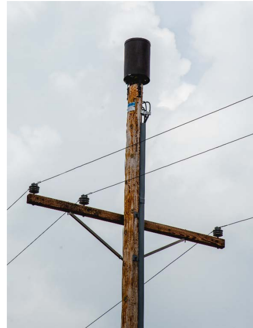
Small cell antenna
