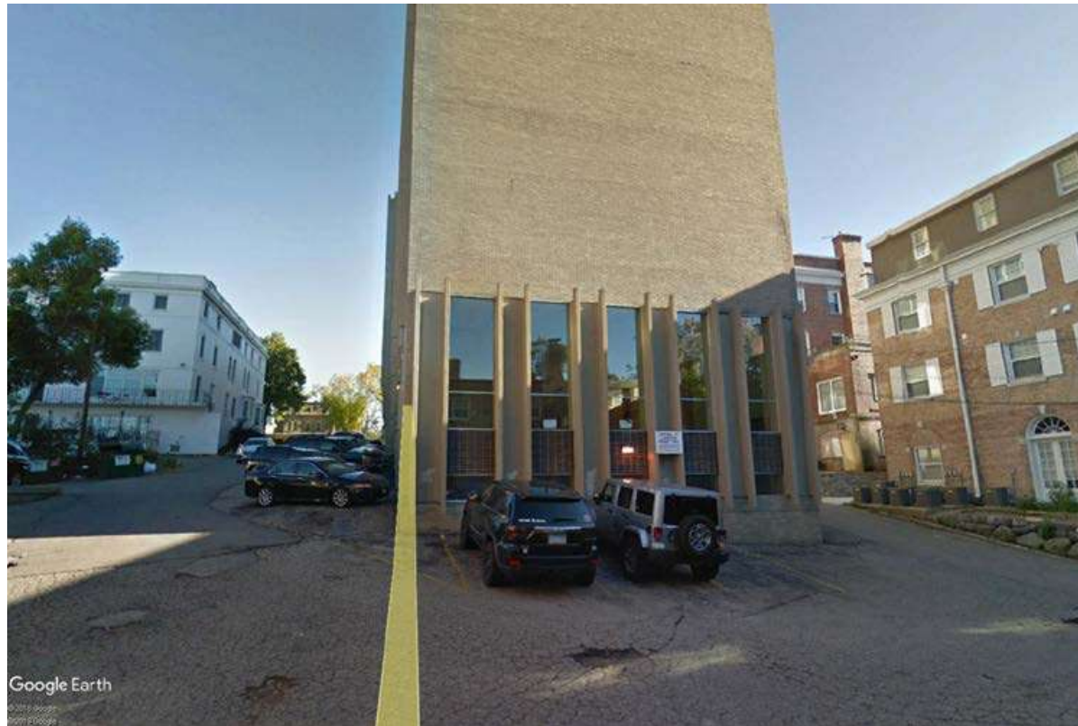
EXISTING SITE, LOOKING SOUTH
