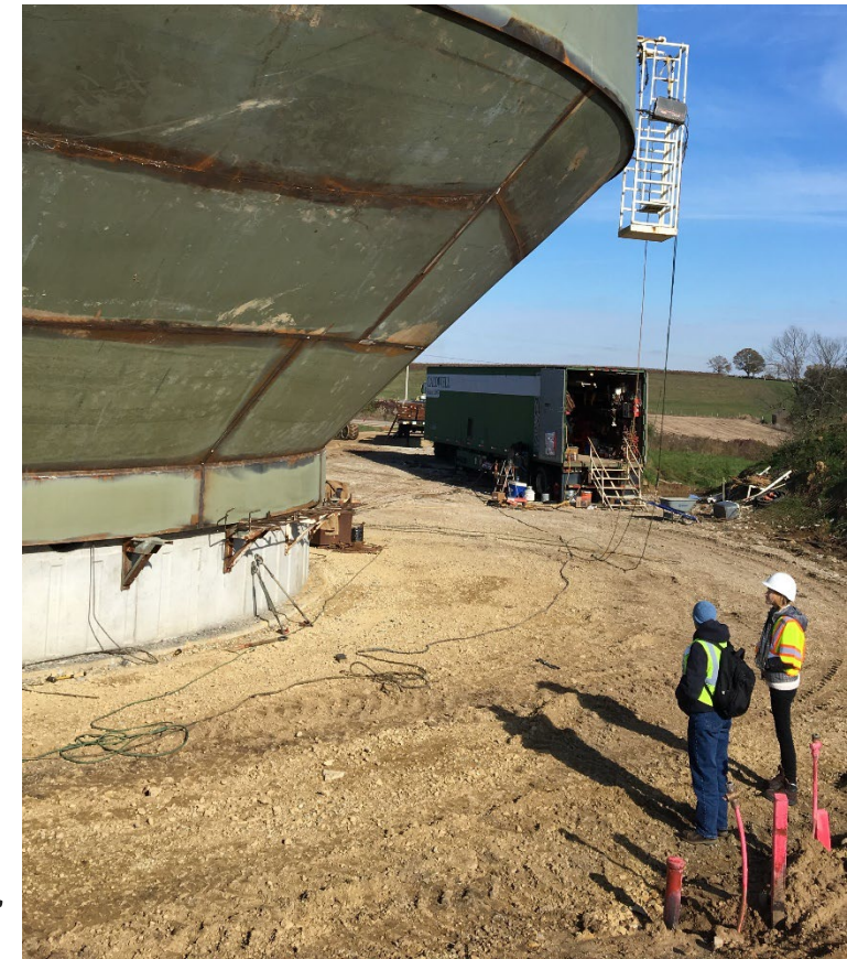
Photo: Construction of a 1M gallon water tower
