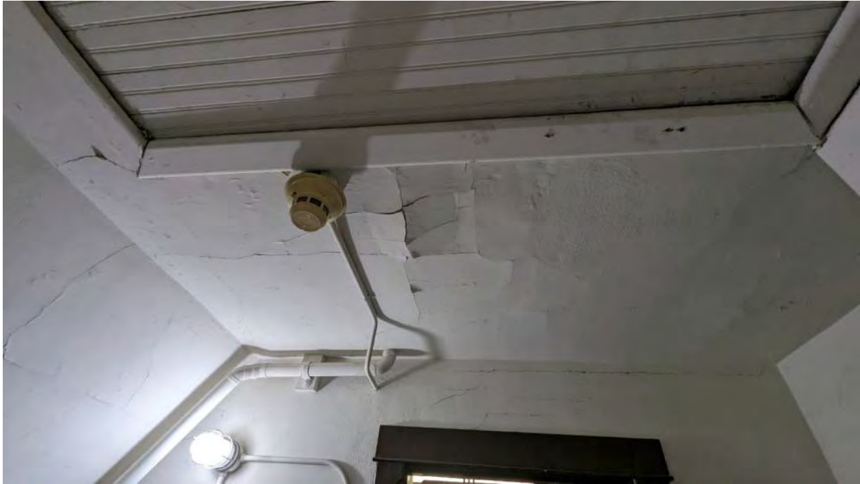
Photo 5: Minor cracking of stair ceiling.
