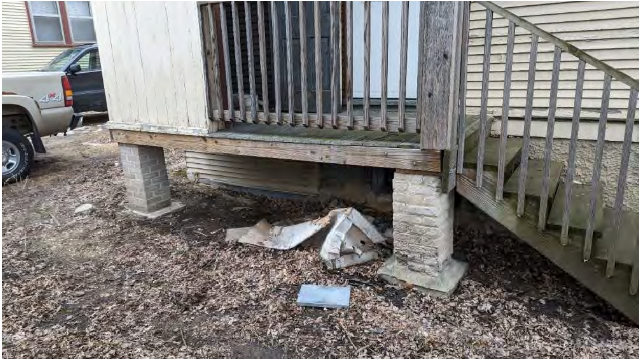
Photo 8: Rear decking supported by masonry columns with minor spalling.
