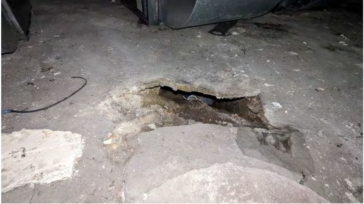
Photo 2: Large hole in basement's concrete slab-on-grade.
