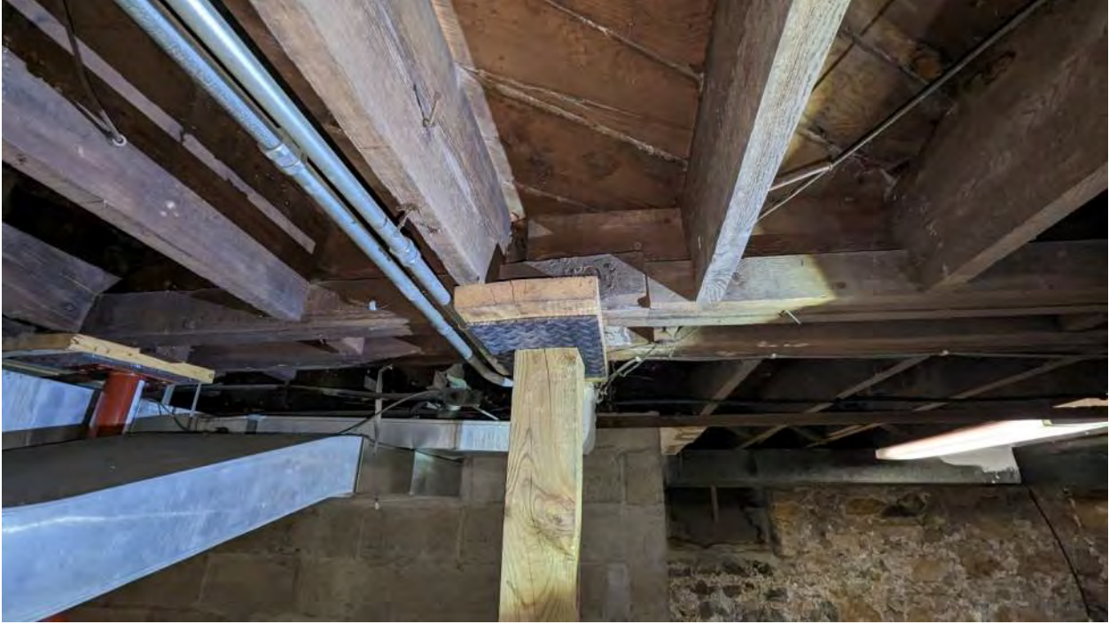
Photo 3: Unsecured temporary shoring in basement.
