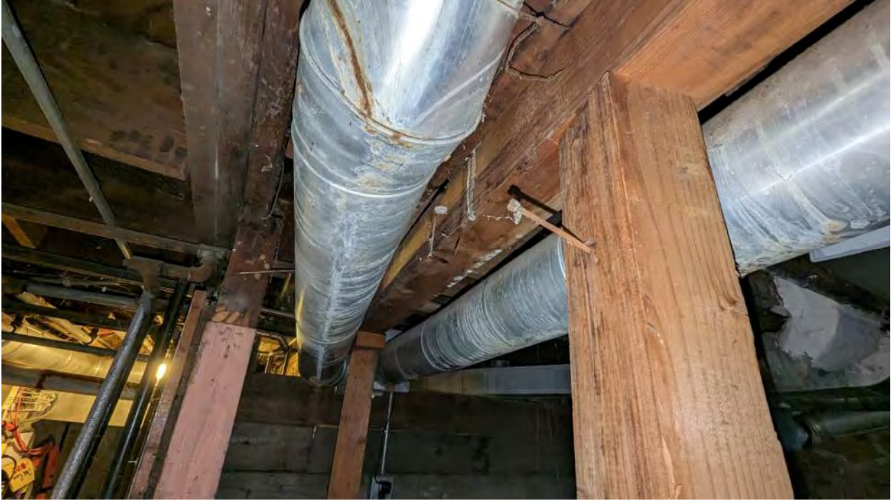
Photo 4: Unsecured temporary wood shoring in basement.
