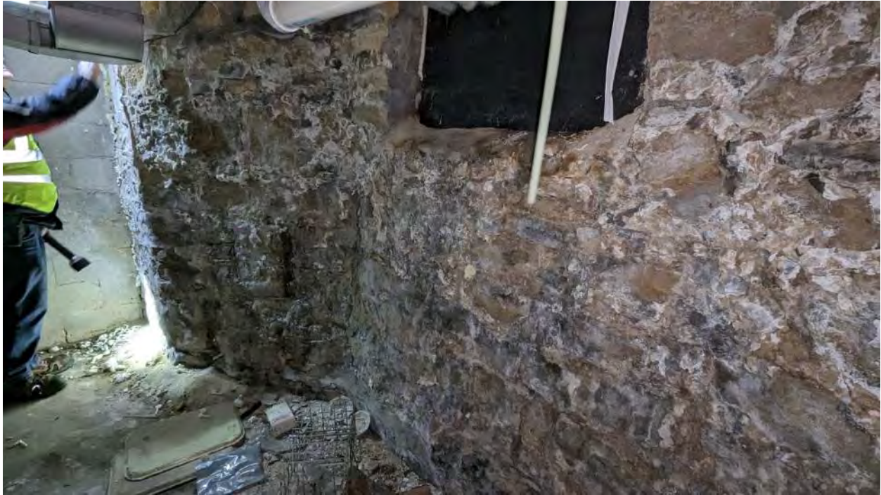
Photo 1: Stone foundation with moderate deterioration on south side of building
