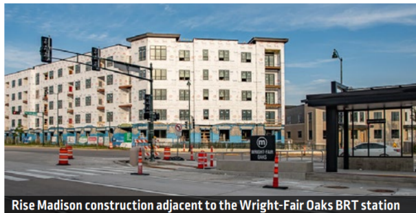
Rise Madison construction adjacent to the Wright-Fair Oaks BRT station
