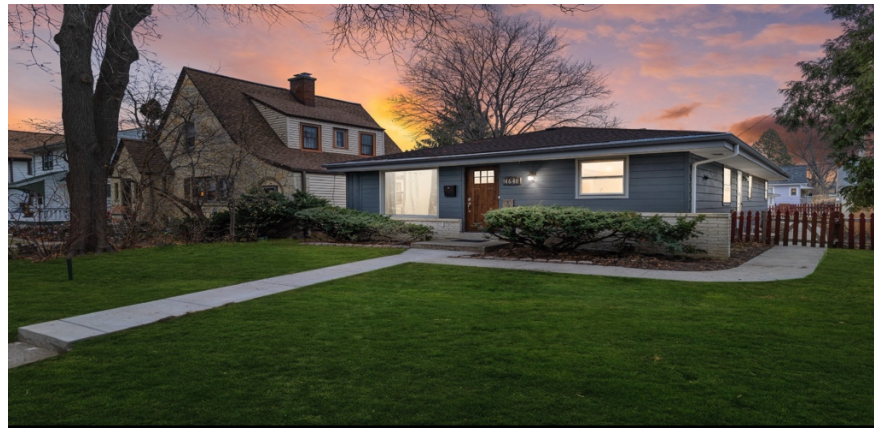
Photos of the last three homes Jason has rehabbed in the city of Milwaukee. Each receiving over $45,000 in renovation.
