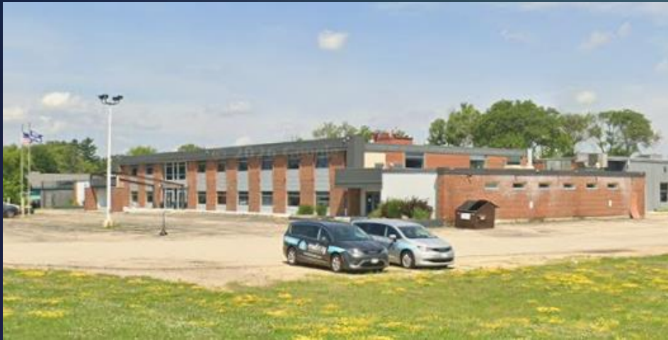
Data Center, East Broadway, Madison WI
