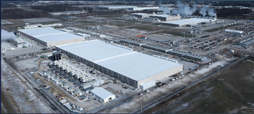
Google Data Center, Council Bluffs IA (datacenters.google)
