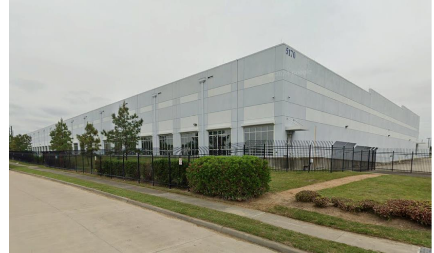
80,000 sq. ft. Data Center, Houston, TX (Google Street View)
