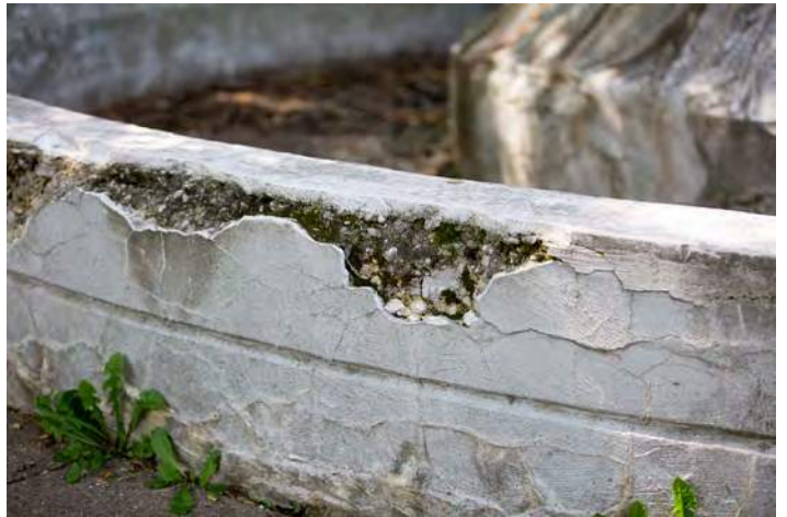
Figure 24: Coarse ring aggregate concrete at lower perimeter
