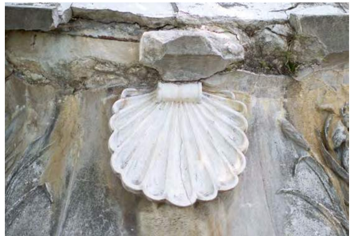
Figure 45: View of damage to limestone at base and relatively intact condition of shell motif
