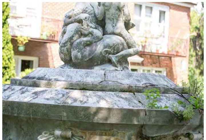
Figure 28: Close up of primary area that should be used when recreating the stone base
