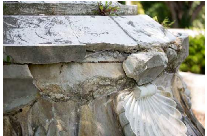
Figure 42: View of damage at tension ring
