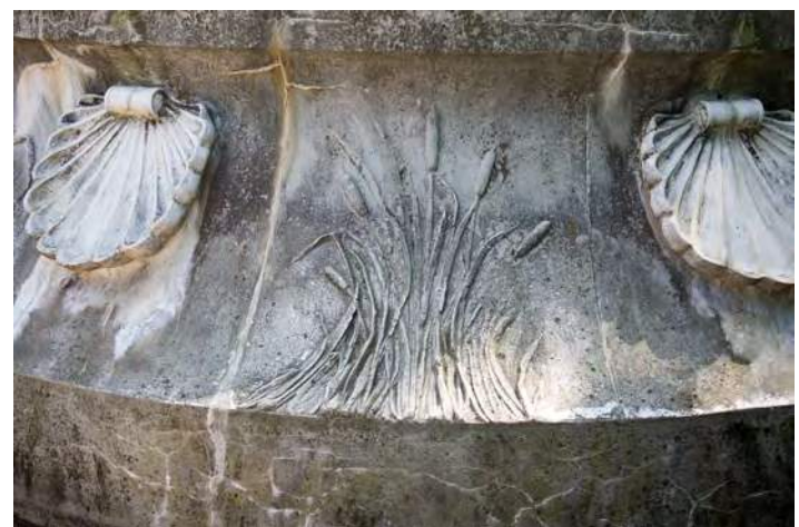
Figure 34: Relatively intact stone to concrete transition
