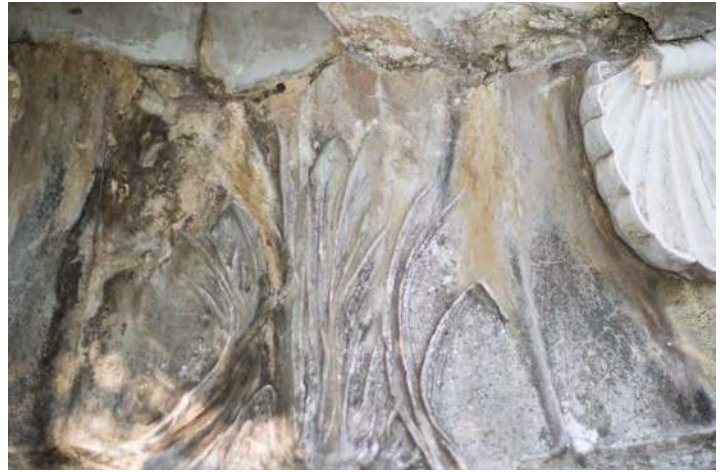
Figure 53: View of degraded material at cattail motif
