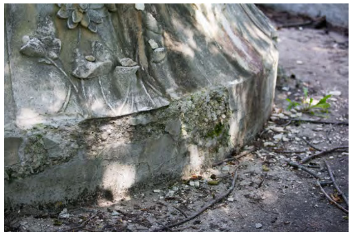
Figure 31: Stone to concrete transition
