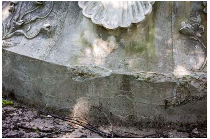
Figure 32: Degradation and mineral staining at trailing water
