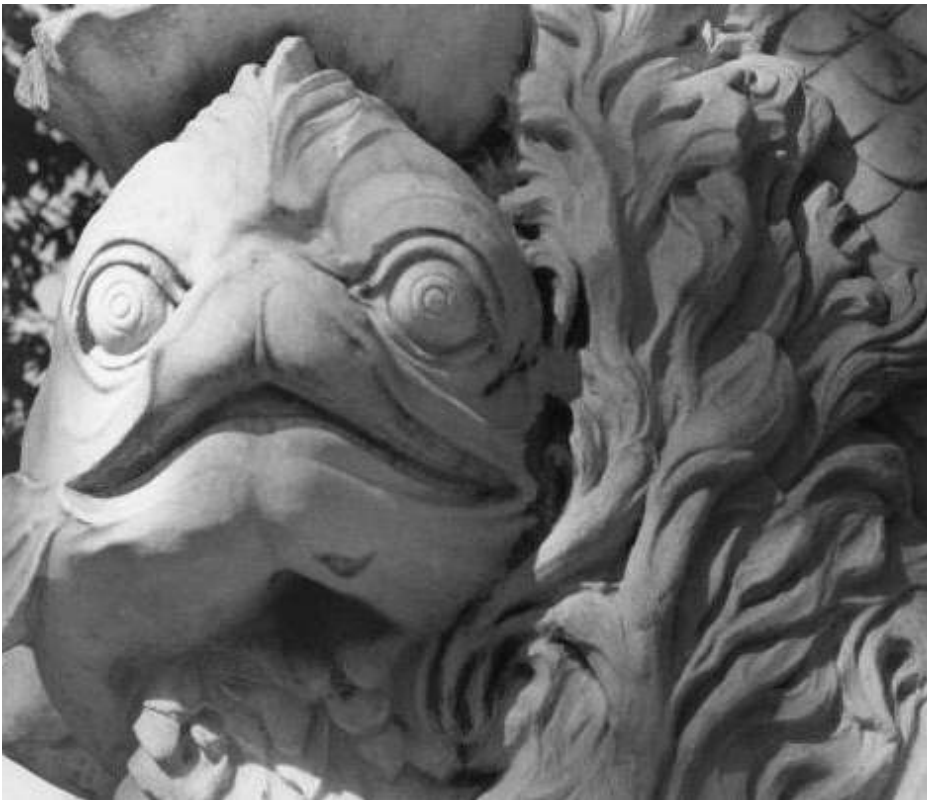
Dolphin in 1973 - The detail evident in this image is exceptional. While unconfirmed, it is apparent that the sculpture was either recently cleaned prior to this photograph or was benefited by a more proactive cleaning and maintenance program. When compared to a contemporary image of the same details it is evident that a significant amount of organic material obscures the detail. A proper conservation cleaning will help to ascertain what, if any, additional damage the piece has suffered.
