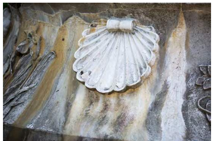
Figure 37: Shell motif condition amid mineral deposits at trailing water
