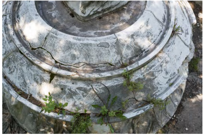
Figure 8: Upper view of pedestal and base - note damage to pedestal has been repaired and appears to have stabilized
