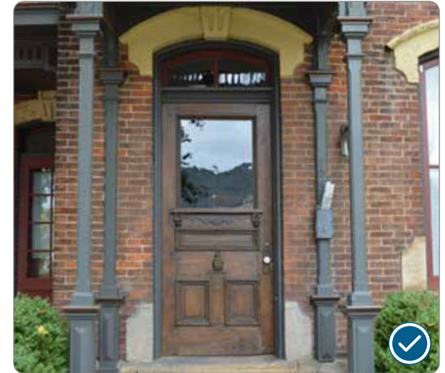
Figure 71: Example of a historic door (41.25.5.d.1).
