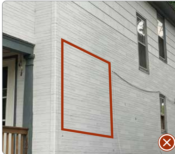
Figure 45: Incompatible replacement of historic siding (41.25.1.b.1).
