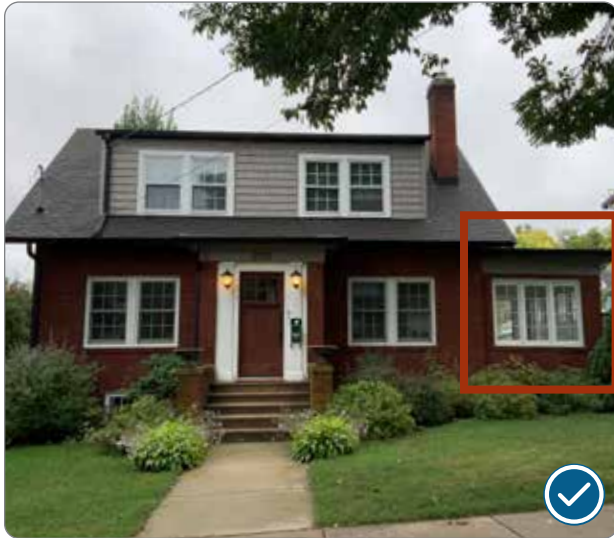
Figure 102: Addition windows that are compatible with the historic building at 1707 Madison Street (41.26.5.1.a-b).
