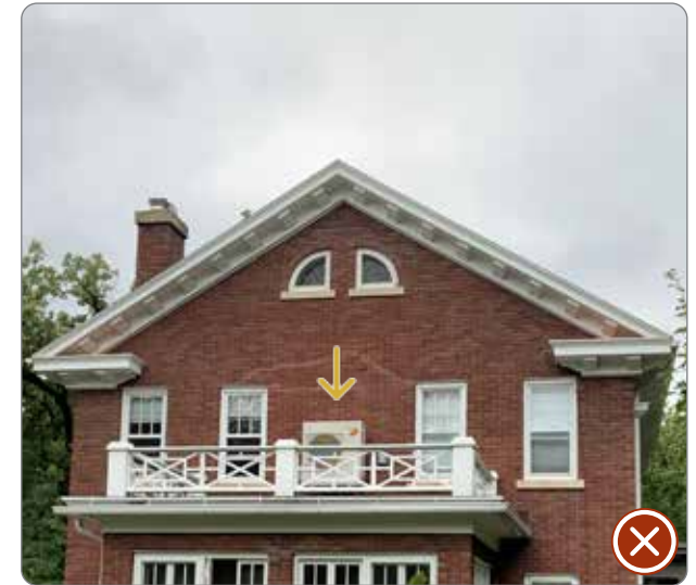
Figure 116: Mechanical equipment on front elevation of residence (41.26.7.1.2).
