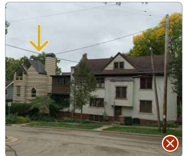
Figure 131: Infill construction demonstrating incompatible wall material (41.27.3.a.1).
