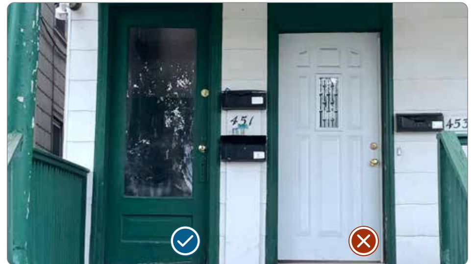
Figure 62: Historic door (on left) and a modern replacement (on right) (41.25.5.a.3).
