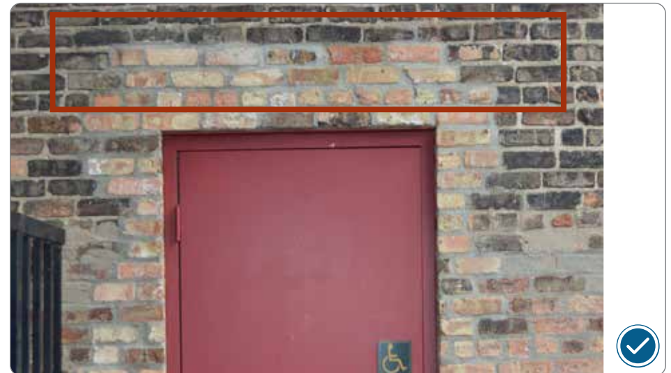
Figure 53: Brick masonry units installed around new accessibility door; the new bricks are currently cleaner than the original (41.25.3.a.3).
