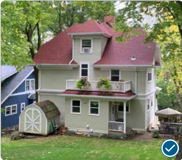
Figure 112: Compatible rear balcony addition at 826 Van Hise Avenue (41.26.6.b.1).
