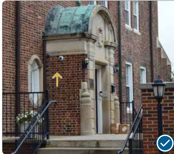
Figure 119: Unobtrusive security camera in Mansion Hill Historic District (41.26.7.c.2).
