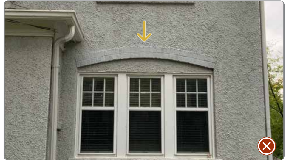
Figure 63: Infilled head above windows (41.25.5.b.1).
