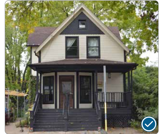
Figure 77: Example of full-width porch enclosed with lattice and with painted handrails at 1380 Williamson Street (41.25.6.b.2-4).
