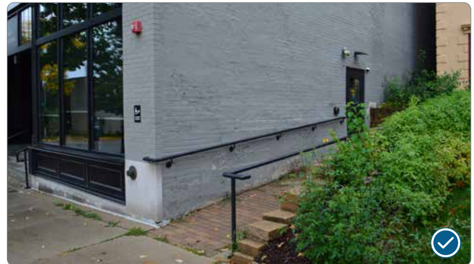
Figure 90: Compatible accessibility ramp to side elevation of 409 E Main Street when primary entrance isn't possible (41.26.1.c.1).
