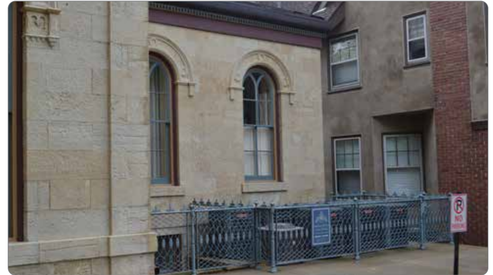
Figure 140: Mechanical equipment screened with fencing from the developed public right-of-way (41.27.7.a.1).
