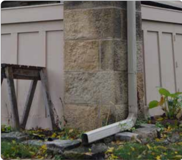
Figure 12: Downspout extension leading water away from building foundation (41.23.2.a.1).
