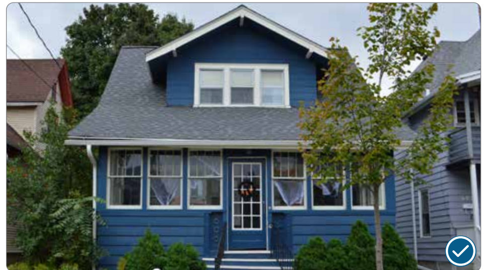
Figure 80: Enclosed porch at 606 S Baldwin Street (41.25.6.c.1).
