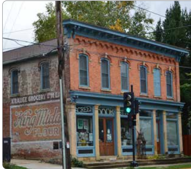
Figure 9: High Integrity Building - 853 Williamson Street.
