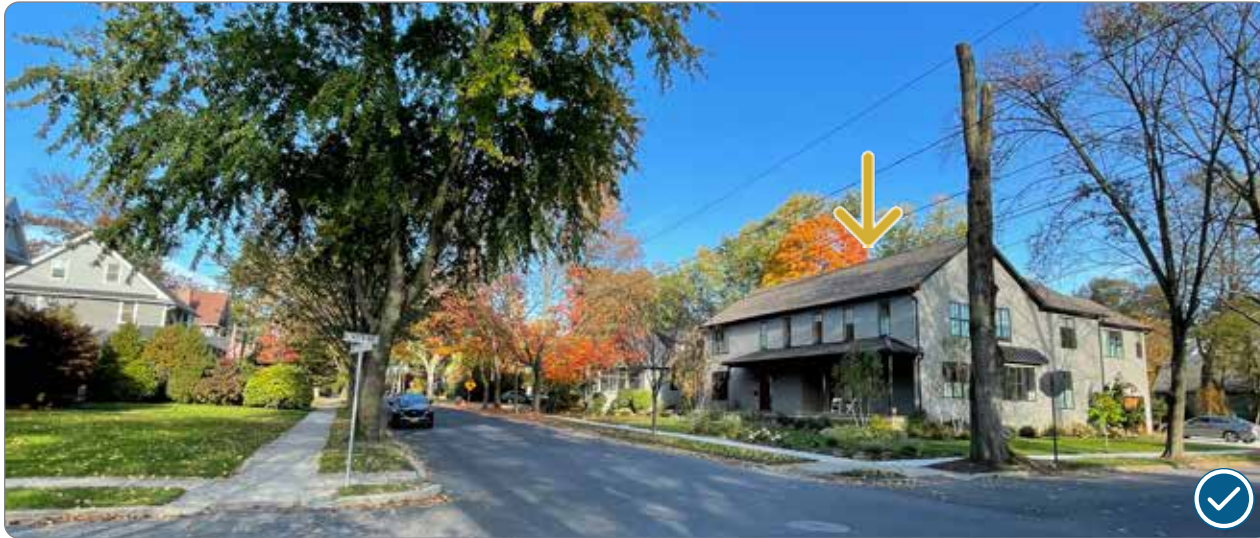
Figure 129: Infill construction demonstrating compatible wall material (41.27.3.a.1).
