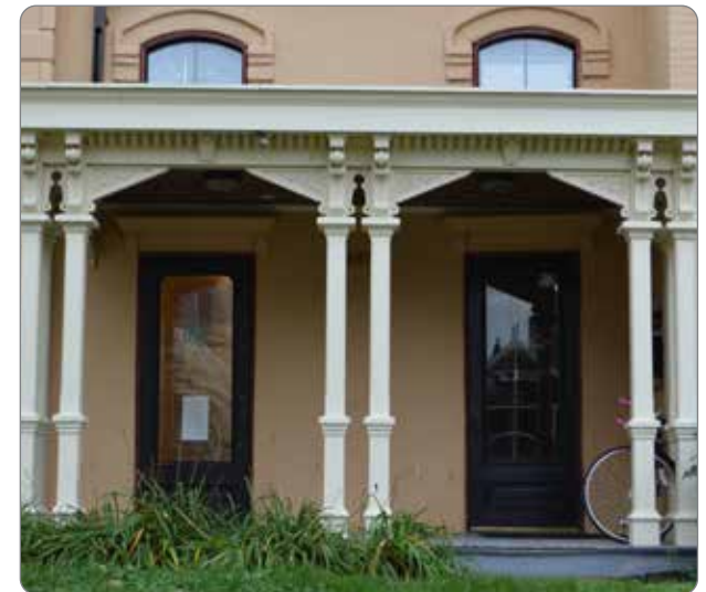
Figure 40: Wood porch details in good condition (41.24.2.b.1).
