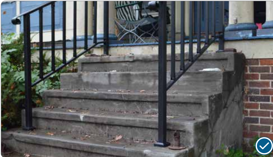
Figure 56: Compatible substitute metal railing replacement (41.25.3.c.1).
