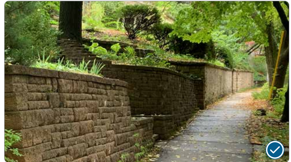
Figure 51: Retaining wall in the University Heights District.
