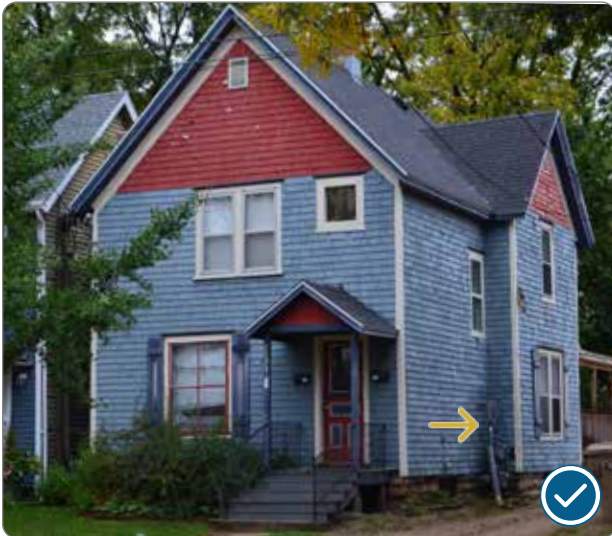
Figure 81: Painted mechanical equipment on side of 1129 Williamson Street (41.25.7.a.2).
