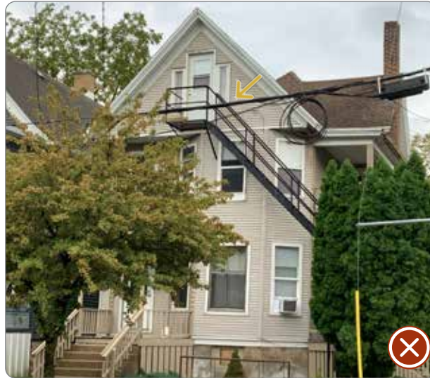
Figure 109: Example of a second exit stairway off the front of the building (41.26.6.a.4).
