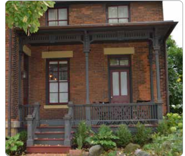
Figure 30: Well preserved porch at 754 Jenifer Street (41.23.6.a.1).
