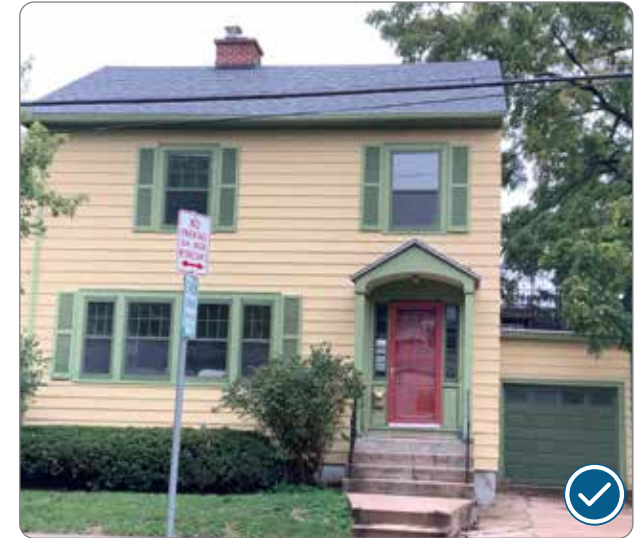
Figure 107: Compatible garage doors that share architectural qualities with the main building at 1005 Oakland Avenue (41.26.5.d.1).
