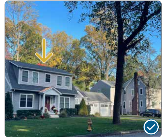
Figure 130: Infill construction demonstrating compatible wall material (41.27.3.a.1).
