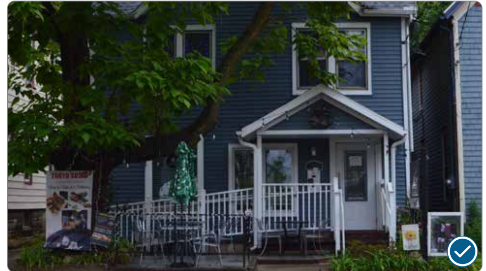
Figure 48: Compatible accessibility ramp constructed to access the primary building entrance at 1133 Williamson Street (41.25.1.d.1).
