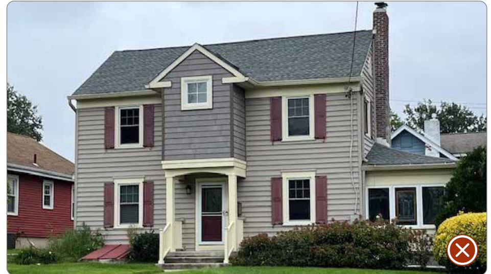
Figure 87: Incompatible front addition on a residential building (41.26.1.a.1).
