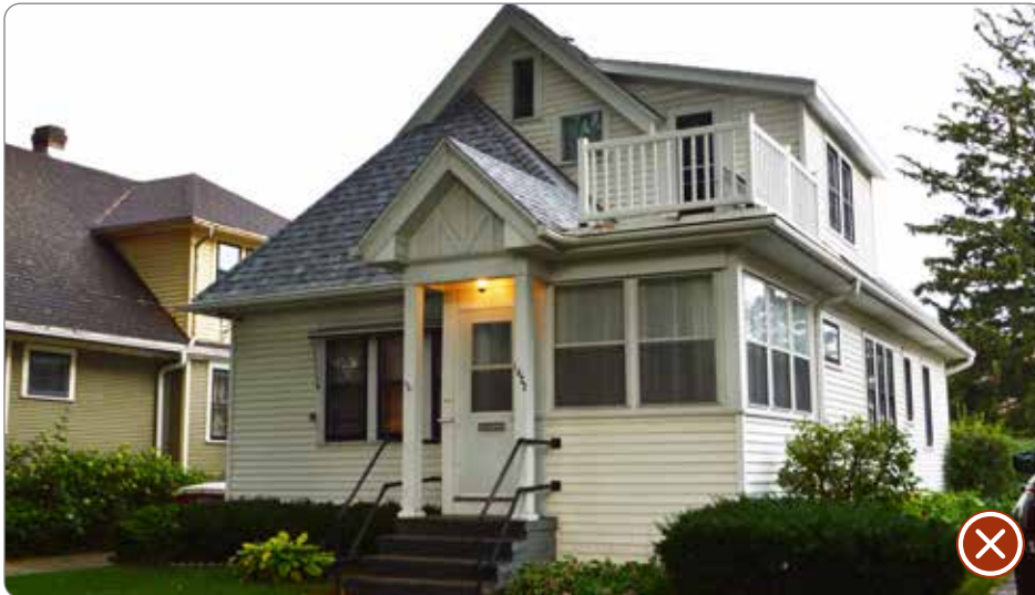
Figure 138: Incompatible front balcony addition (41.27.6.b.1).
