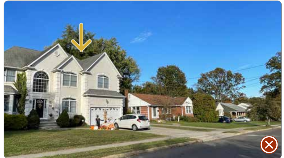
Figure 125: Infill construction demonstrating incompatible architectural expression and massing (41.27.1.a.5).
