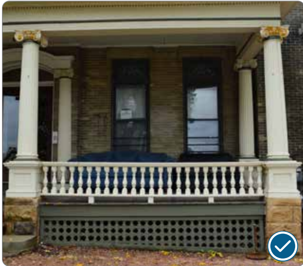
Figure 75: Example of a porch with compatible details and lattice for ventilation (41.25.6.b.3).
