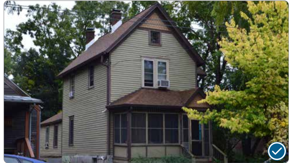
Figure 79: Enclosed porch that retains historic elements 1121 Williamson Street (41.25.6.c.1).
