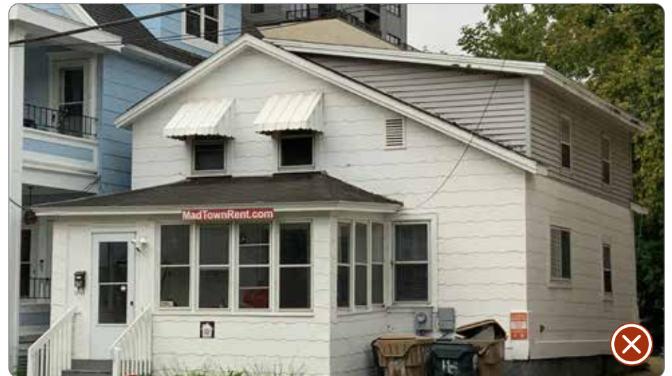
Figure 101: Incompatible dormer addition to residence (41.26.4.f.1-4).
