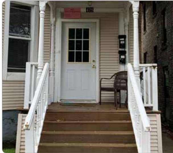
Figure 33: Porch flooring and steps replaced with compatible substitute material similar in visual qualities.
