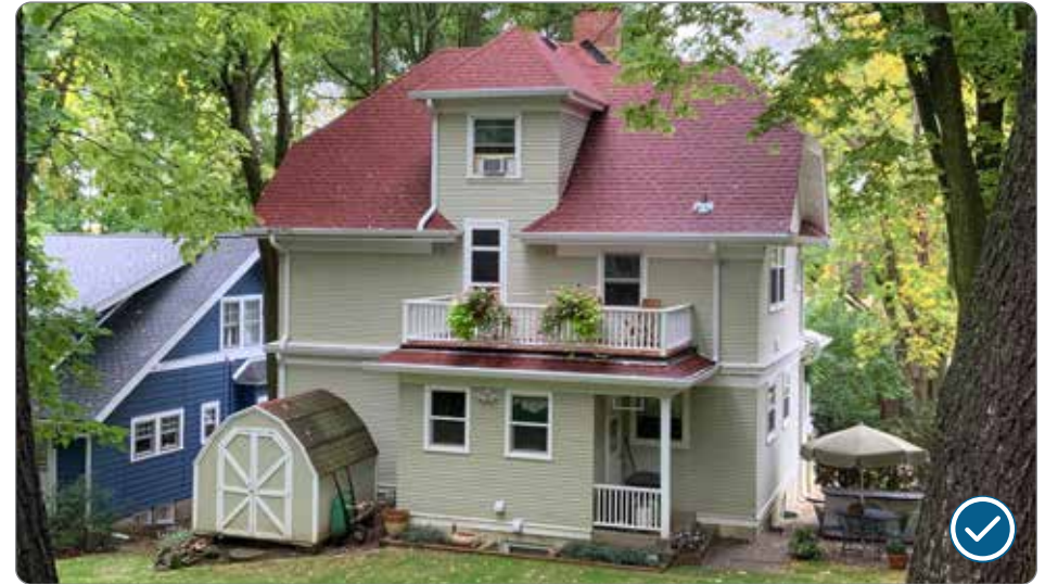
Figure 89: Compatible rear addition at 1826 Van Hise Avenue (41.26.1.b.1).
