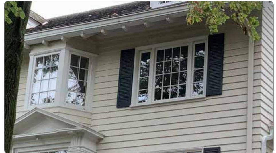
Figure 66: Replaced divided light windows (41.25.5.c.3).
