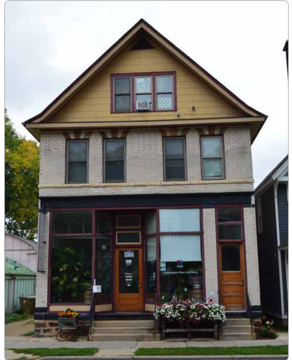
Figure 1: Example of well maintained building in the Third Lake Ridge Historic District at 1014 Williamson Street.
