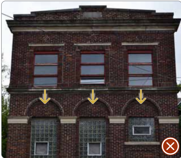
Figure 44: Infill of historic openings on masonry building (41.25.1.b.1).
