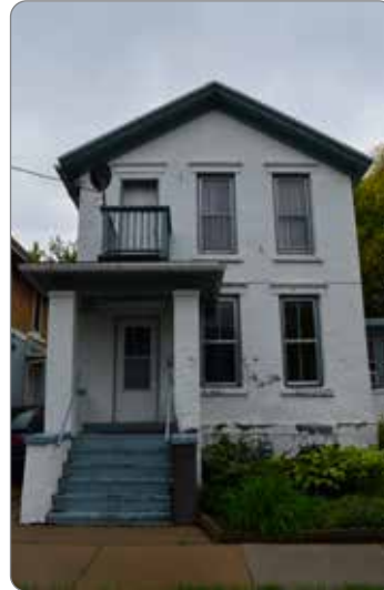
10 South Franklin Street
