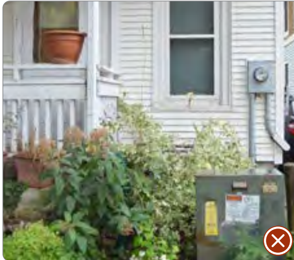
Figure 82: Utilities at the front of a building, in this placement, it should be screened with fencing or landscaping (41.25.7.a.2).
