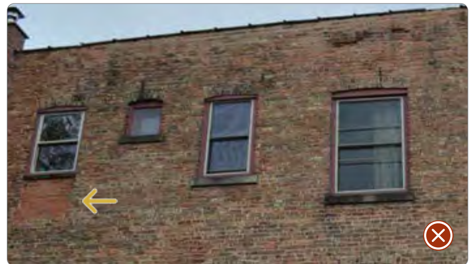
Figure 64: Adjusted sill height (41.25.5.b.3).
