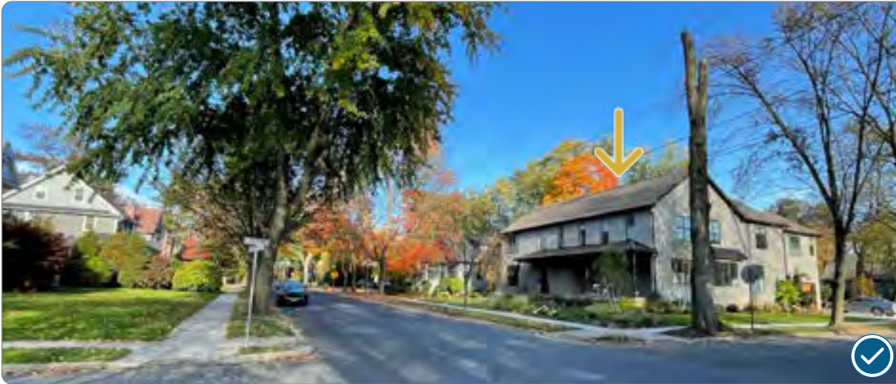
Figure 129: Infill construction demonstrating compatible wall material (41.27.3.a.1).
