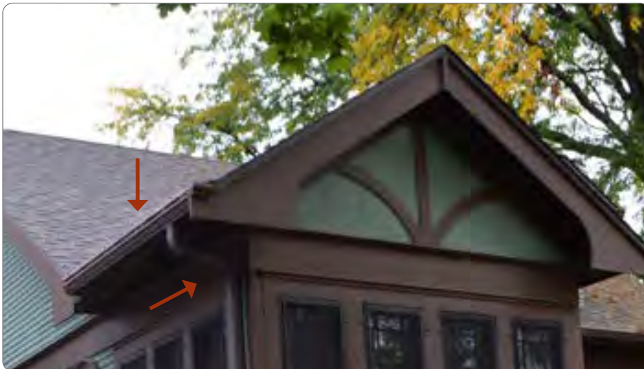
Figure 23: Example of a gutter guard protecting gutter system at 1520 Rutledge Street (41.23.4.a.1).
