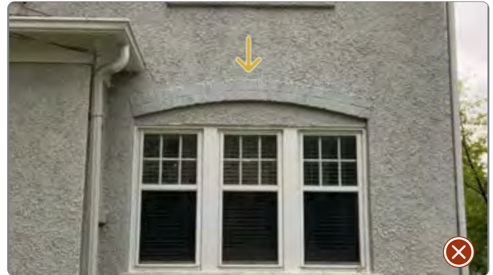
Figure 63: Infilled head above windows (41.25.5.b.1).
