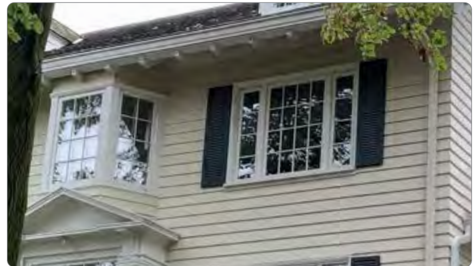
Figure 66: Replaced divided light windows (41.25.5.c.3).
