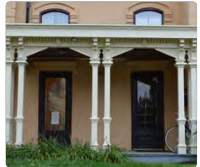
Figure 40: Wood porch details in good condition (41.24.2.b.1).
