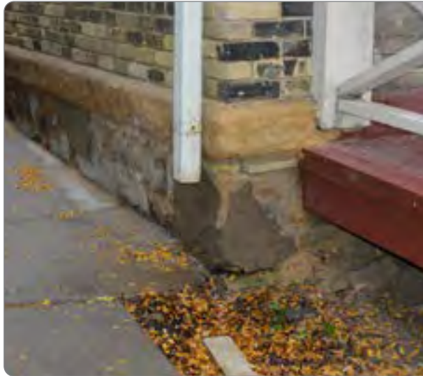
Figure 13: Improper drainage gutter system resulting in deterioration of foundation walls (41.23.2.a.1).
