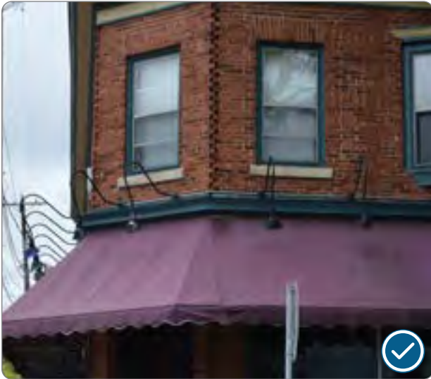
Figure 118: Commercial decorative lighting (41.26.7.c.1).
