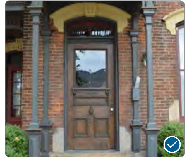
Figure 71: Example of a historic door (41.25. 5.d.1).
