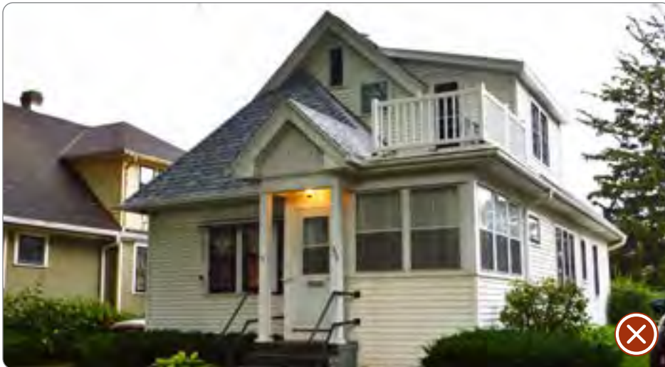
Figure 138: Incompatible front balcony addition (41.27.6.b.1).
