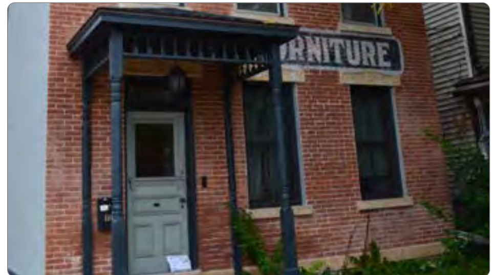
Figure 74: Example of a historically accurate entrance (41.25. 6).
