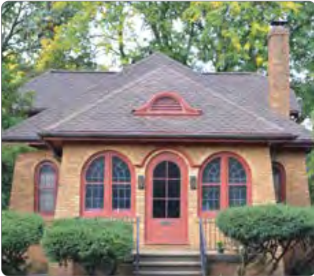
Figure 8: High Integrity Building - 624 S Thornton Avenue.
