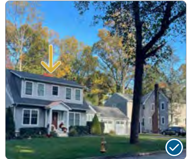
Figure 130: Infill construction demonstrating compatible wall material (41.27.3.a.1).
