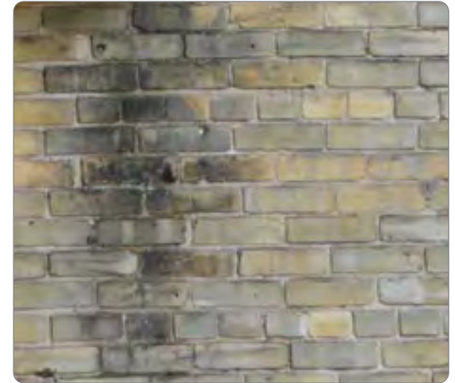
Figure 15: Dirty masonry that can be cleaned without a Certificate of Approval (41.23.3.a.1).
