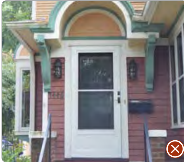
Figure 106: Incompatible storm door, new storm doors need to be full light (41.26.5.d.1).
