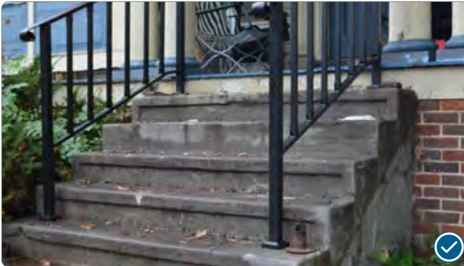
Figure 56: Compatible substitute metal railing replacement (41.25.3.c.1).
