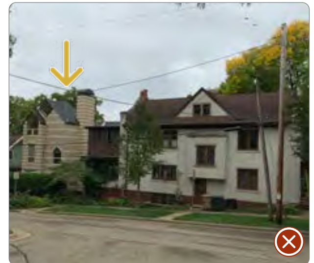
Figure 131: Infill construction demonstrating incompatible wall material (41.27.3.a.1).
