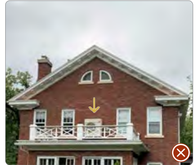
Figure 116: Mechanical equipment on front elevation of residence (41.26.7.1.2).
