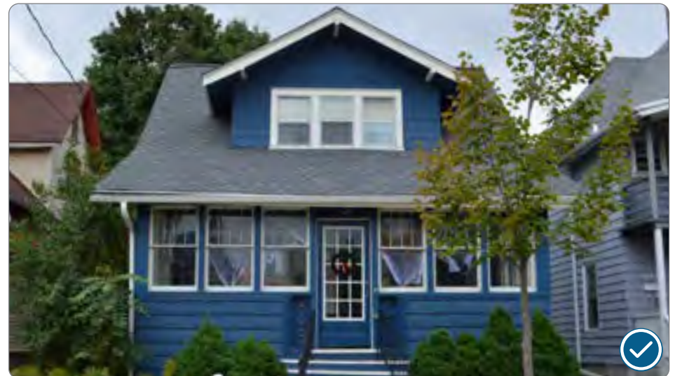
Figure 80: Enclosed porch at 606 S Baldwin Street (41.25.6.c.1).
