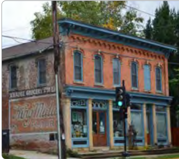
Figure 9: High Integrity Building - 853 Williamson Street.
