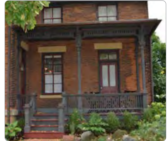
Figure 30: Well preserved porch at 754 Jenifer Street (41.23.6.a.1).
