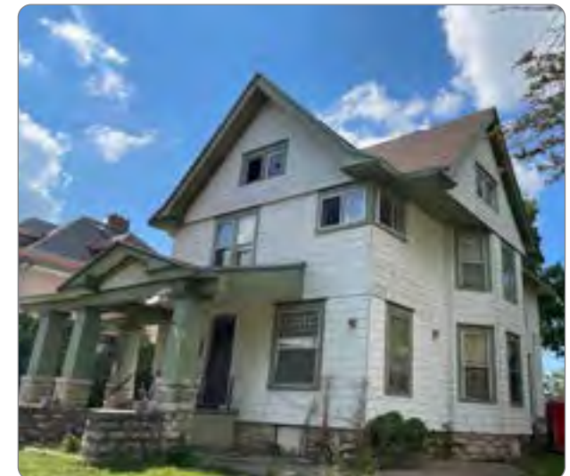
Figure 11: Low Integrity Building.
