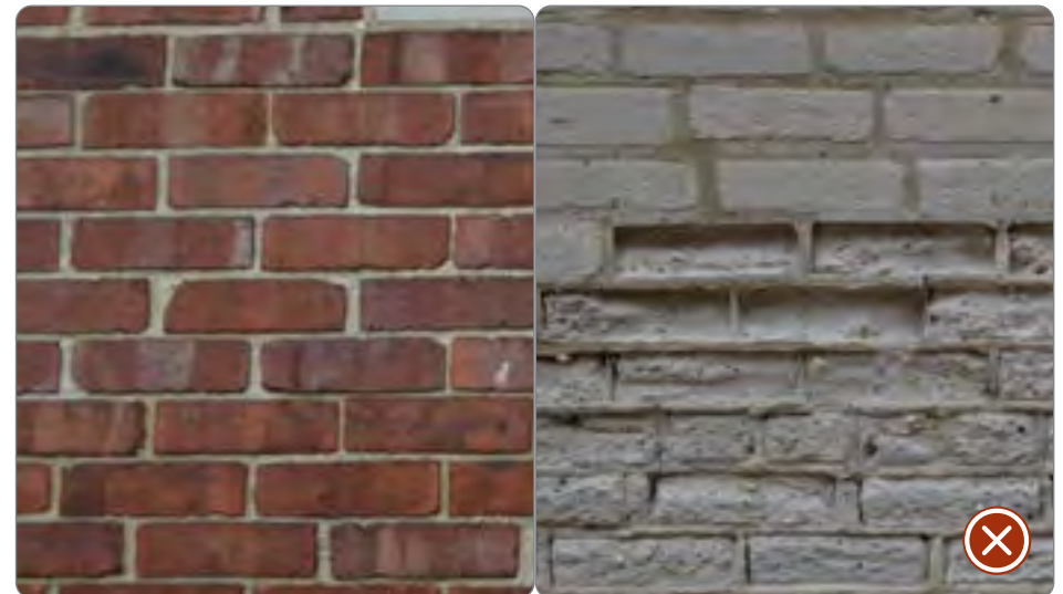
Figure 38: Proper vs. improper mortar alterations (41.24.2.a.1).
