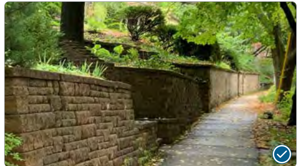
Figure 51: Retaining wall in the University Heights District.
