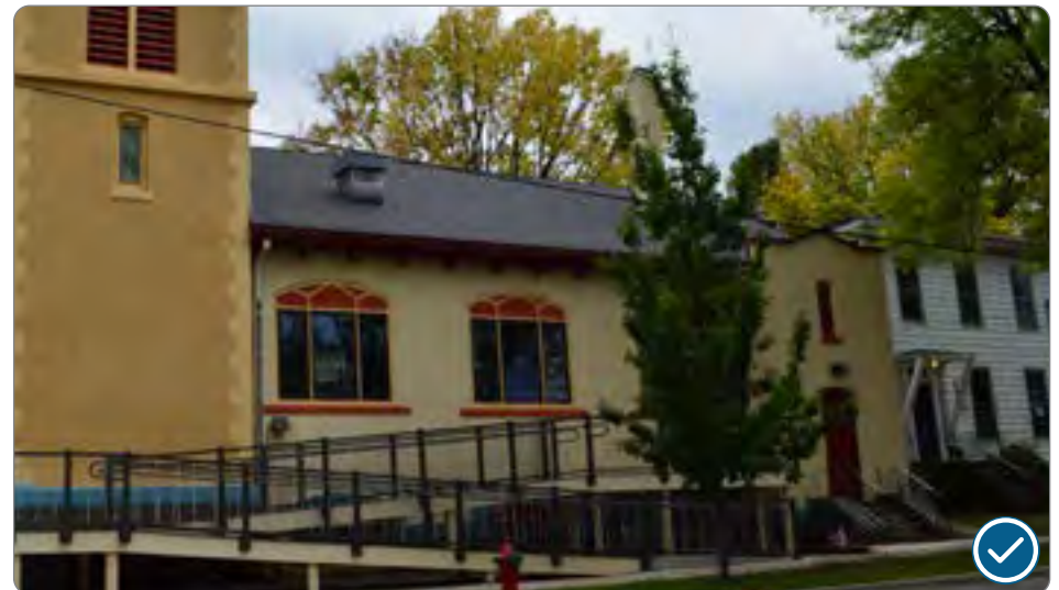
Figure 49: Compatible accessibility ramp constructed on side of historic public building at 504 S Brearly Street (41.25.1.d.2).
