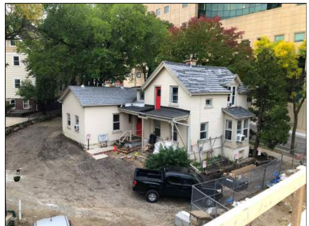
EXISTING BUILDING FROM REAR OF SITE
