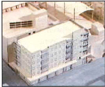
Figure 8: View of neighborhood retail residential building at corner of South Butler and East Main Streets
