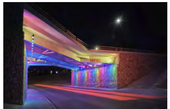
HWY 30 Overpass Lighting
