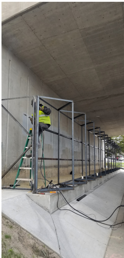
Design by Julia Shilling. Gallas Metalworks detailed, manufactured, and installed 150' of lenticular wall.
