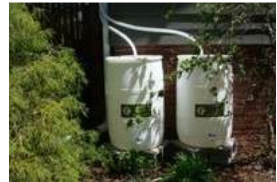
Cisterns and small rain barrels like these may be incorporated for rainwater collection and reuse.
