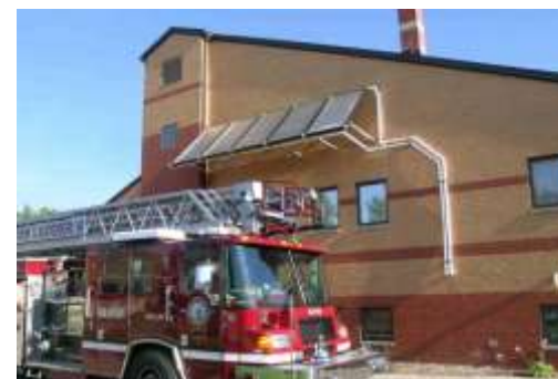
Solar hot water panels on Madison Fire Station 6 provide a good nonresidential example
