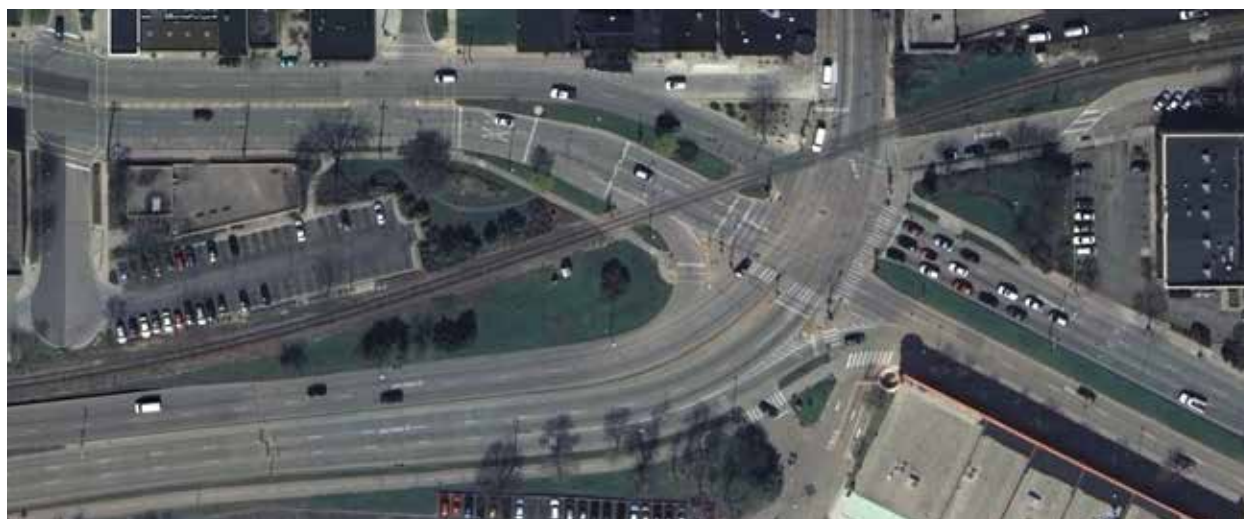
Figure 10. Existing Conditions at the East Gateway
