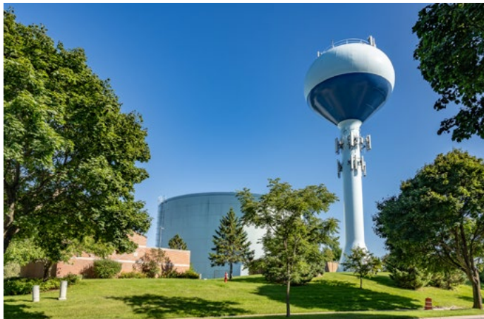
Well 20 serves part of the Southwest Area.
