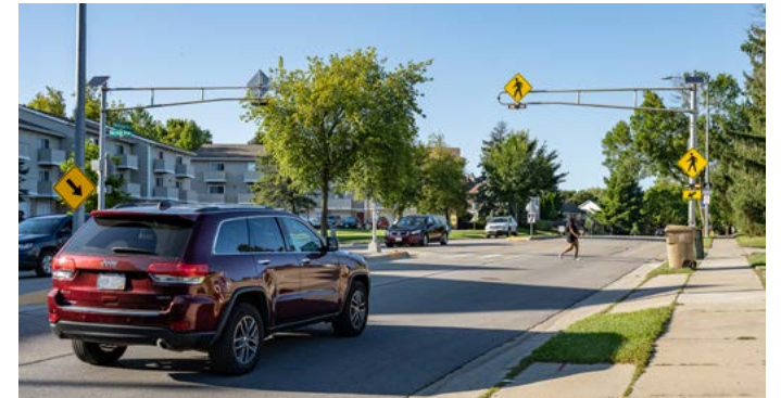
The RRFB at McKenna Boulevard and Morraine View Drive helps pedestrians cross safely. Safe Streets Madison prioritizes improvements like RRFBs on a citywide basis.
