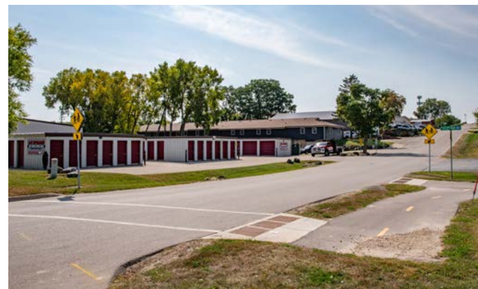
Much of Seybold Road is in the Town of Middleton and lacks sidewalks, curb and gutter, stormwater management, and street trees.
