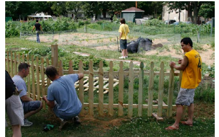
Residents help install a fence around the Meadowood Park Community Garden supported by Southwest Neighborhood Plan CDBG funds
