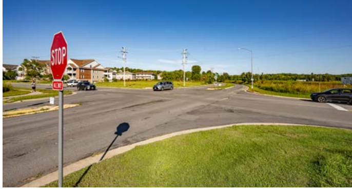
The Maple Grove–Nesbitt–Cross Country intersection is planned for conversion from a four-way stop to a roundabout.
