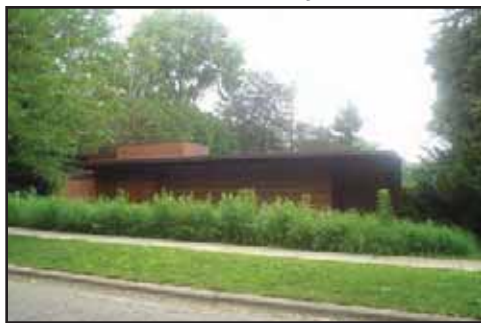
The Jacobs House, a Frank Lloyd Wright Usonian home in the Westmorland Neighborhood
