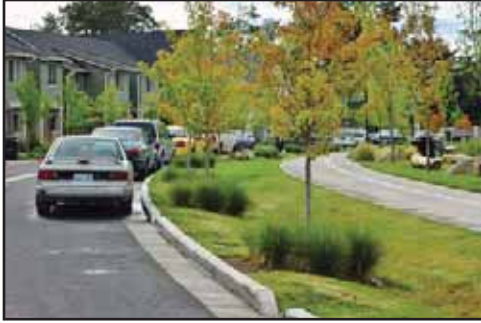
A bioswale in a street terrace helps infiltrate stormwater © 2006 Sitephocus, LLC., www.sitephocus.com
