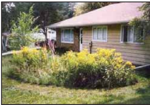
A residential rain garden infiltrates storm water on-site
