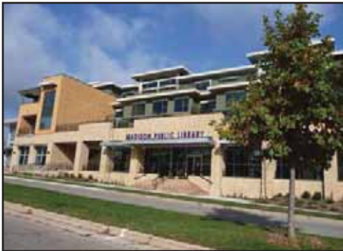
The new Sequoia Branch of the Madison Public Library, part of the Sequoia Commons redevelopment at South Midvale and Tokay Boulevards
