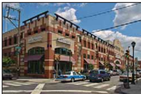
This Whole Foods Market offers parking on the upper level of the building © 2006 Sitephocus, LLC., www.sitephocus.com
