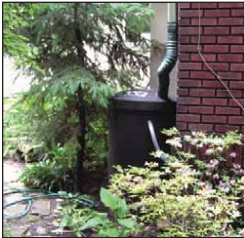
A rain barrel at a private residence stores water for later use
