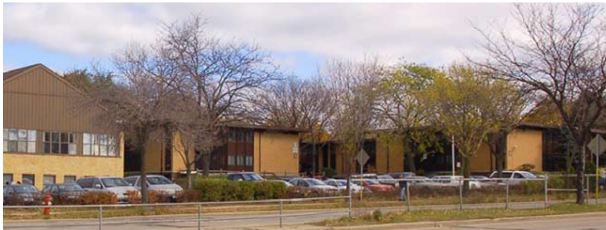
Image 21: Northport Community Learning Center and Northport Apartments.
