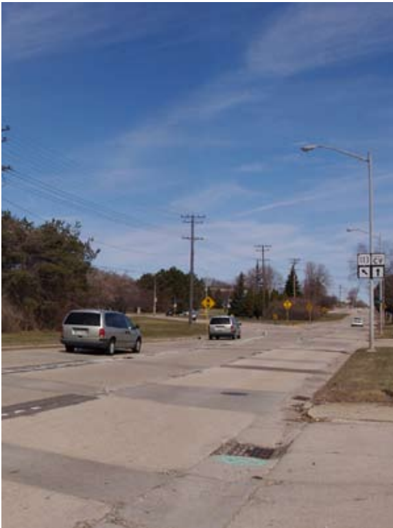
Image 7: Street-level photo of the Northport Drive - Packers Avenue - Highway CV intersection.
