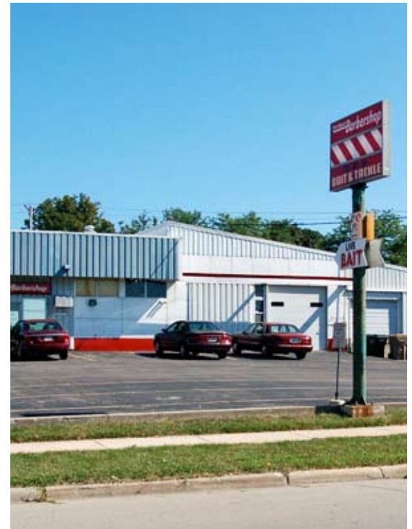
Image 9: Street-level photo of buildings along Troy Drive.
