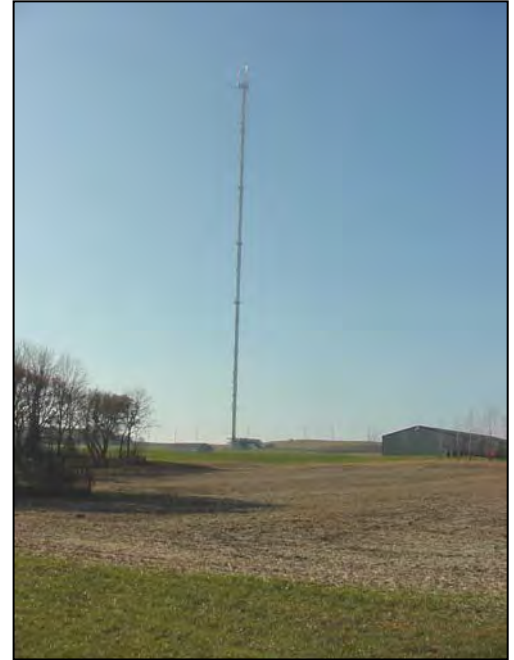
View of telecommunication tower from Mineral Point and Junction Road intersection
