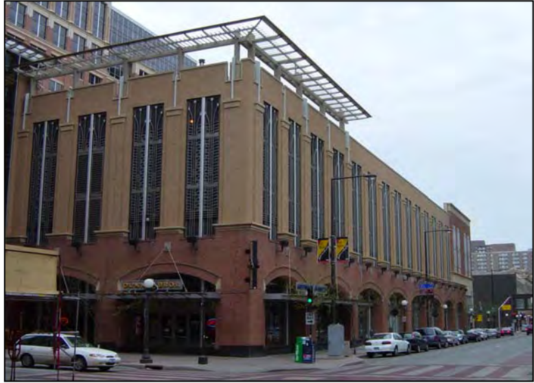
Example of structured parking in mixed-use building with first floor retail. The building design and façade hide the visual presence of the parking structure.
