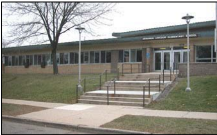
The entrance of Lincoln Elementary School is off Sequoia Trail. Aesthetic improvements, such as new plantings, in front of the building would make it more appealing.
