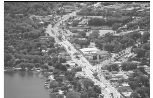
The redevelopment of the 65-acre site from Madison Labor Temple to Morningstar Dairy could provide new retail, office, and housing opportunities.
