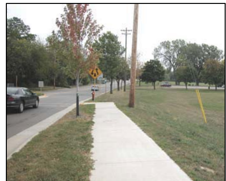
The recent removal of the West Olin Avenue bridge has opened up access to Franklin Field. Sidewalks should be extended along the northern side of Franklin Field.
