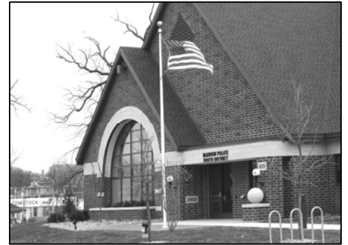
Private and public investments, such as the South Police District Station, continue to stabilize the area.
