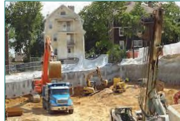
Construction of Brownlofts Apartments, University Avenue, 2013.
