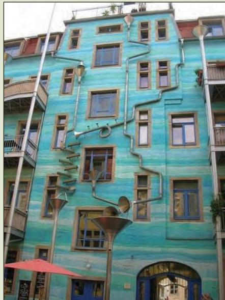
Rain drainage system Dresden, Germany
