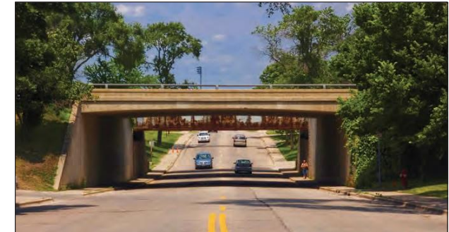
Current view of bridge underpasses
