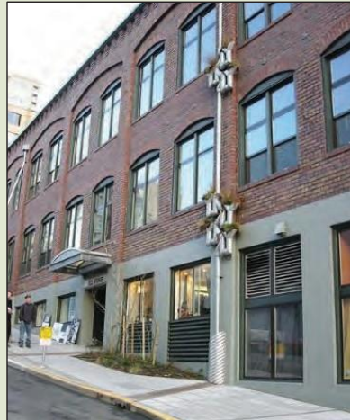
Rain drainage system, Seattle, WA
