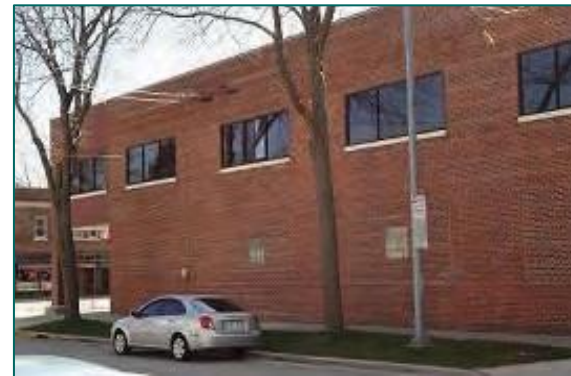
Blank walls lack vi- sual interest and are not pedestrian-friendly. North Paterson Street, Madison.
