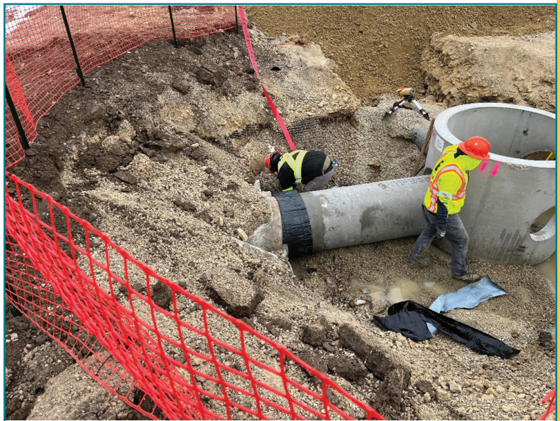
John Nolen Drive Reconstruction
