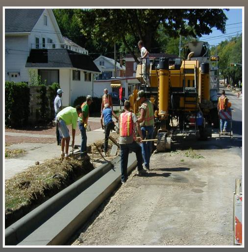
⇒ HAND PLACED C&G VS. MACHINE PLACED C&G
