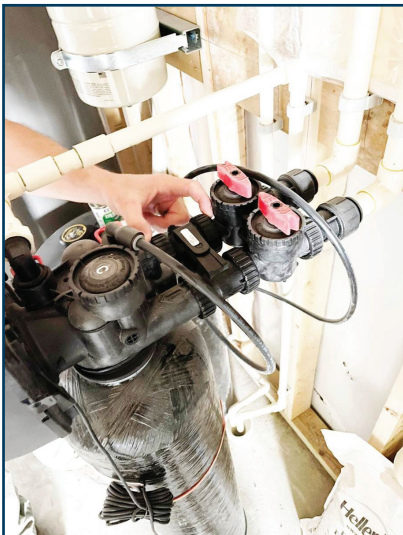
A blending valve is a small component added to the back of a water softener, which allows greater control over home water quality, and environmental benefits.
