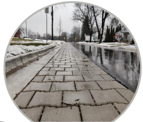
Permeable Pavement installed with GI Study
