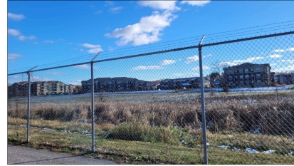
8' GALVANIZED CHAINLINK W/ BARBWIRE (C)
