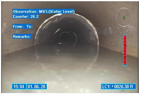
Staining/buildup from groundwater infiltration, gaps and cracks in pipe are common in the area.
