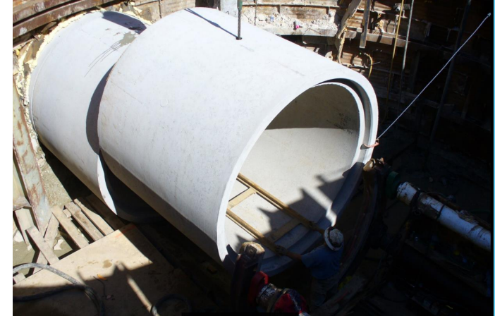
Above: 96" pipe on University Ave (2013) Below: storm sewer inlet on W Doty St
