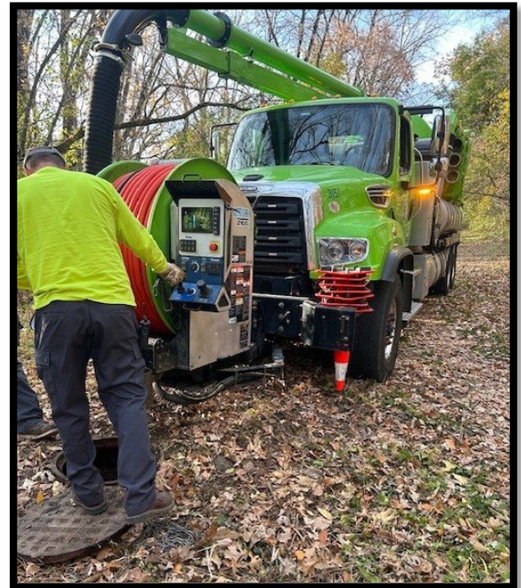
Figure 21 Vactor and crew cleaning sanitary mains via access structure in Sauk Creek greenway
