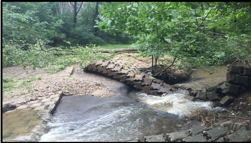
Figure 19 Failed sanitary access path
