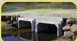
3a - Culverts at sanitary access path crossing - to allow consistent vector access. Culvert will be topped with concrete for stability
