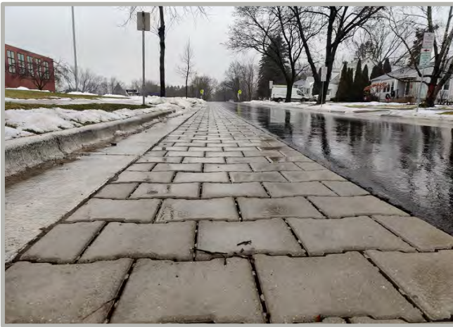
Permeable Pavement installed with pilot project
