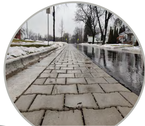
Permeable Pavement installed with GI Study
