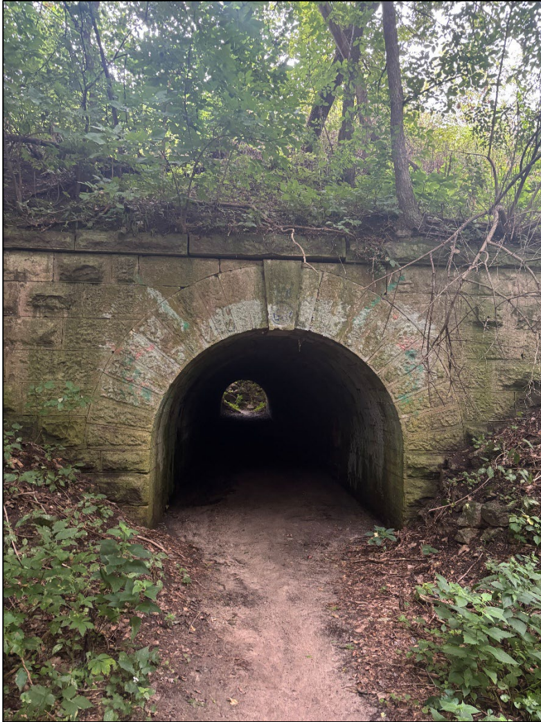
Existing storm pipe (Craig Ave end looking south)
