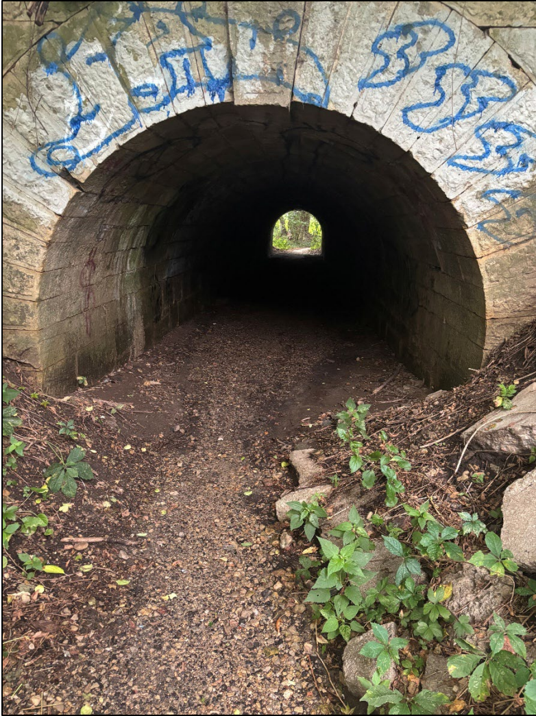
Existing storm pipe "entrance" (Old Middleton Rd end looking north)
