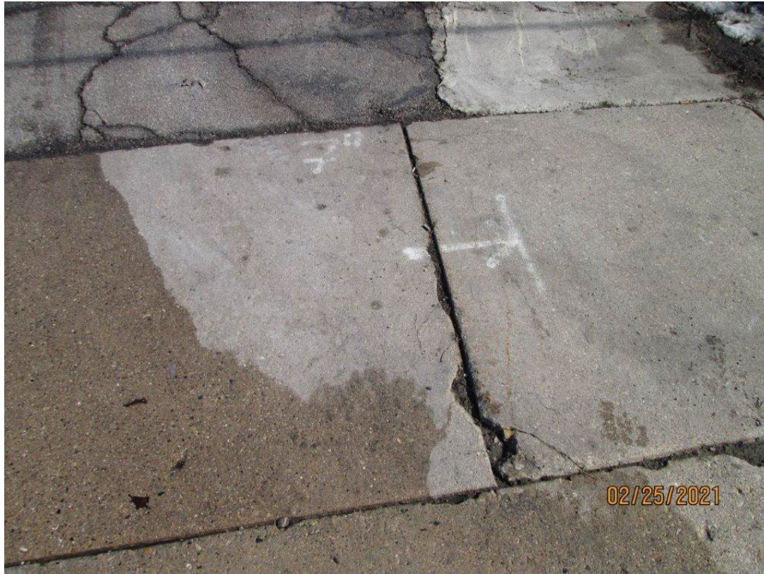
Voids and Erosion of Joints
