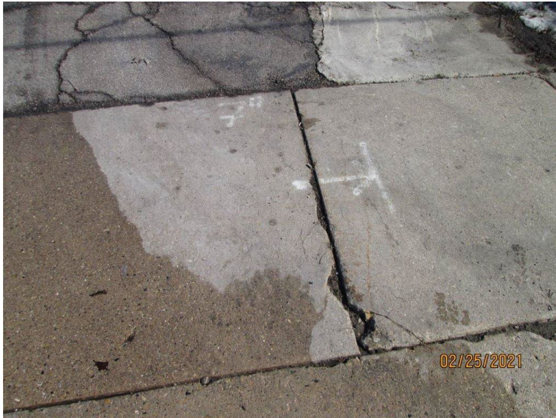
Voids and Erosion of Joints
