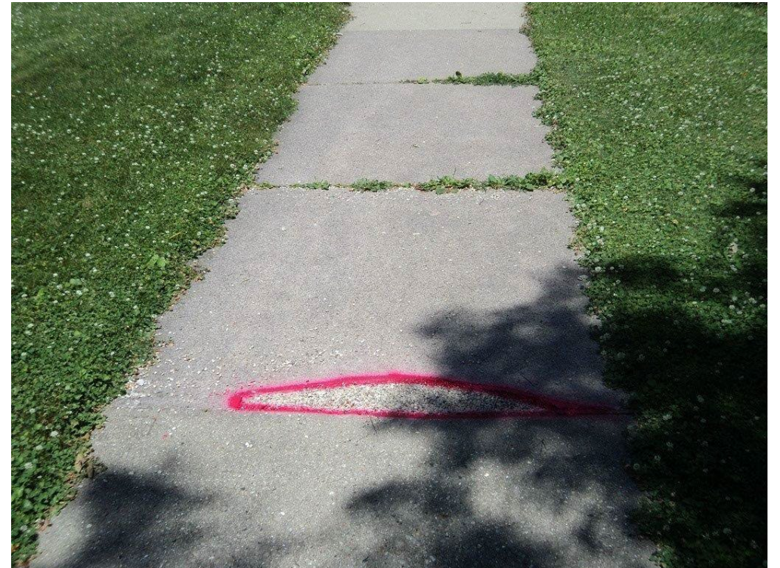
Voids and Erosion of Joints
