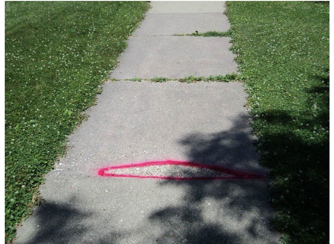
Voids and Erosion of Joints
