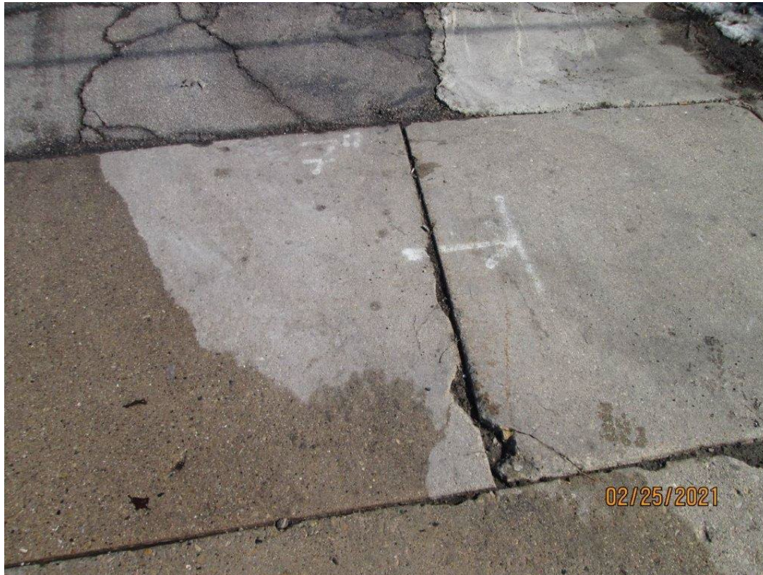
Voids and Erosion of Joints
