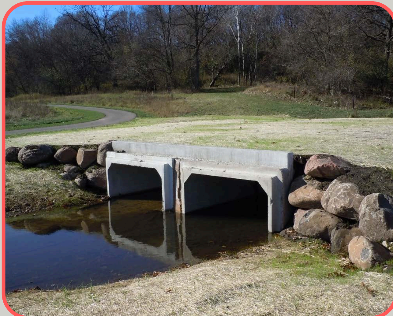
Sanitary access path improved crossing Culverts will help vector truck more safely cross the channel
