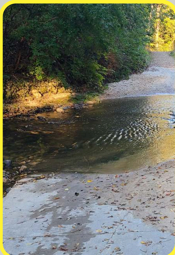
Construction/ Channel Maintenance crossing - Concrete Ford -
