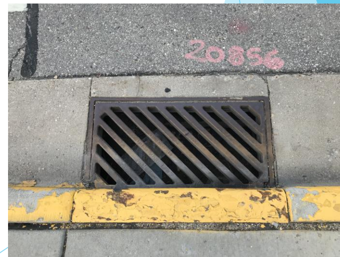
Below: storm sewer inlet on W Doty St
