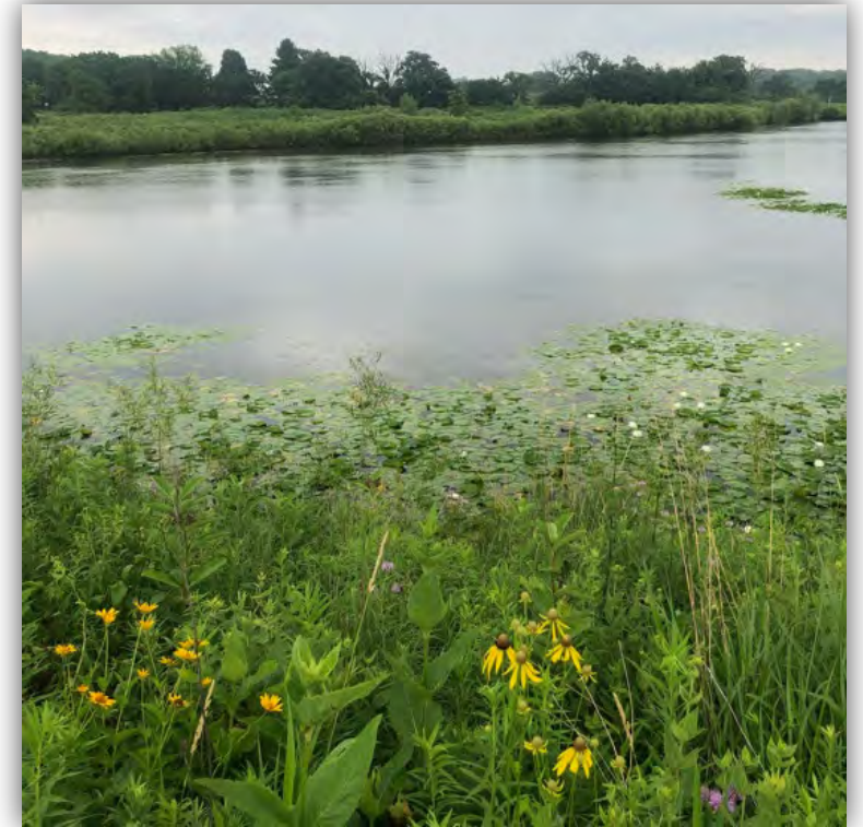
City of Madison Stormwater Utility Retention Pond
