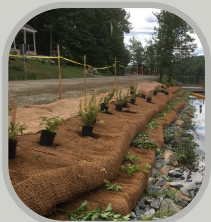
Example of soil lifts used on lake shoreline in Vermont Source: Vermont BioEngineering Manual
