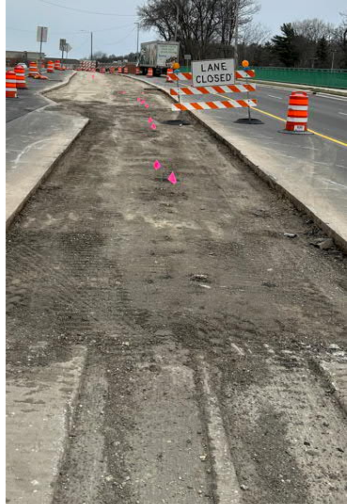
Median Prepared for Curb & Gutter
