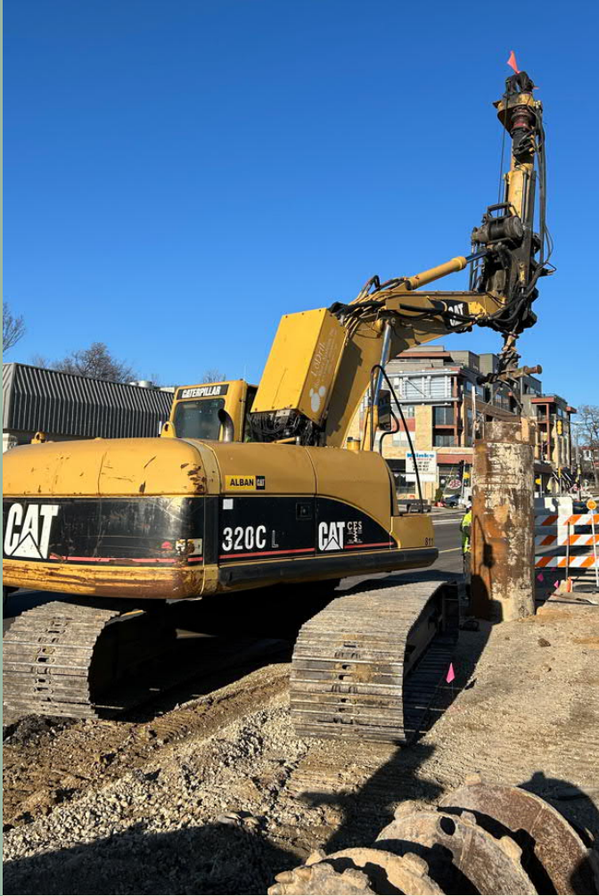
Drilling Overhead Sign Base Shafts
