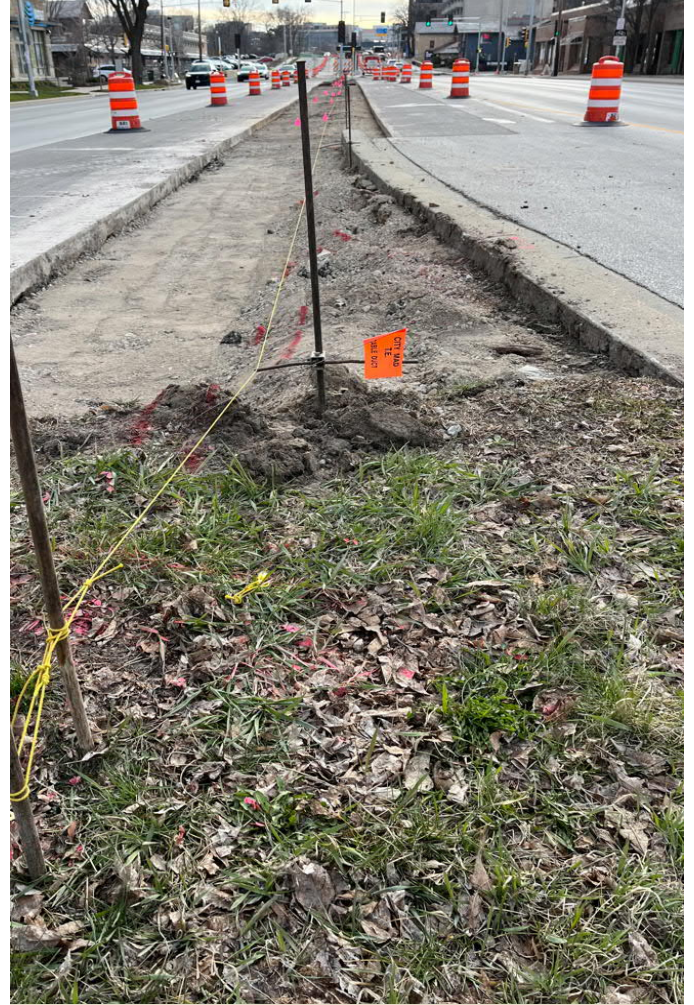
Median Prepared for Curb & Gutter
