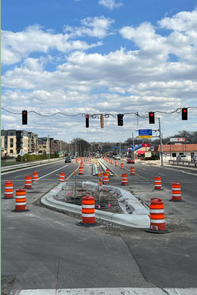
Median Island (Marshall Ct./Ridge St.)
