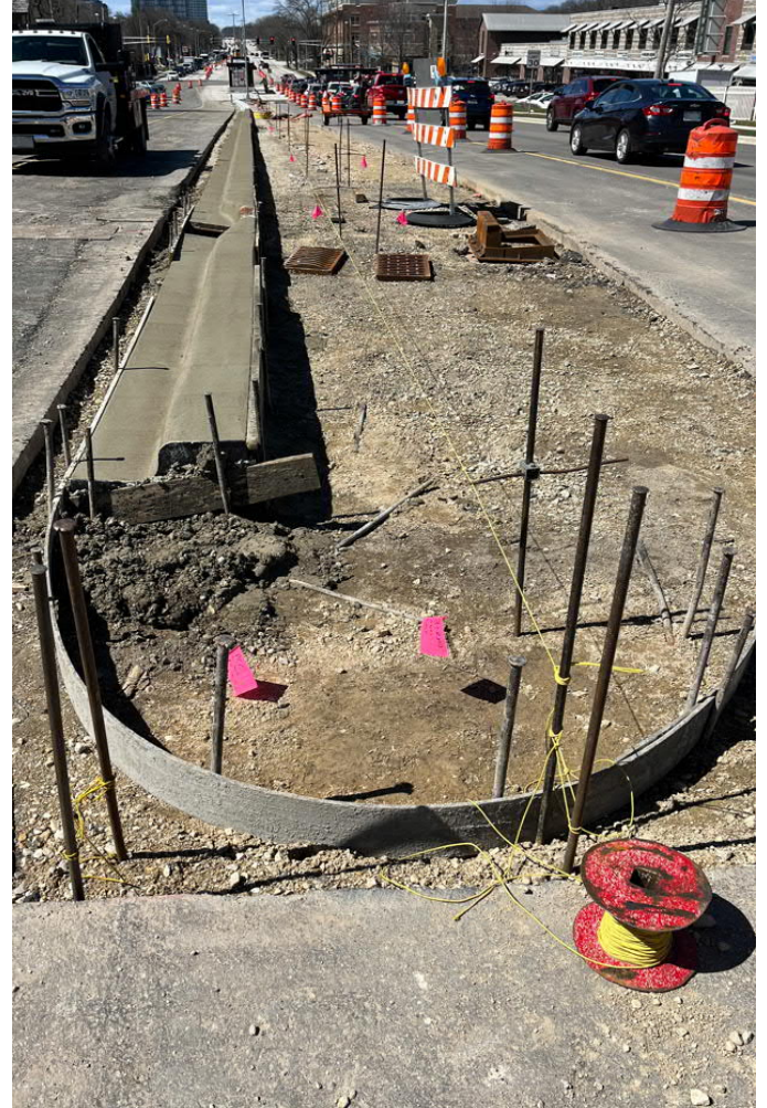
Median Curb & Gutter (West of Schmitt Pl.)
