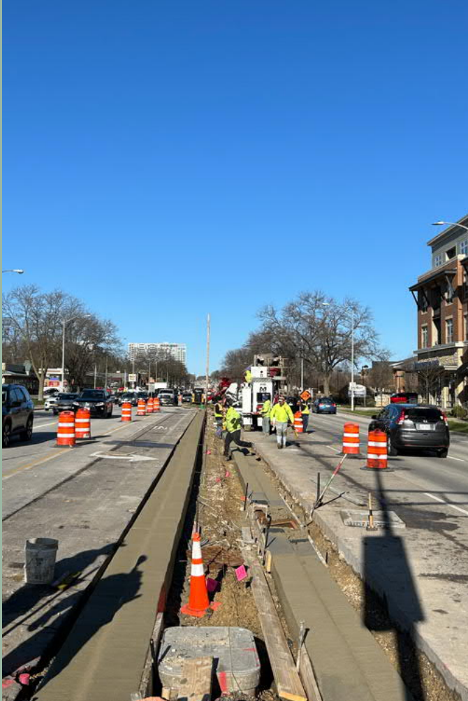
Median Curb & Gutter (West of Hill St./Shorewood Blvd.)
