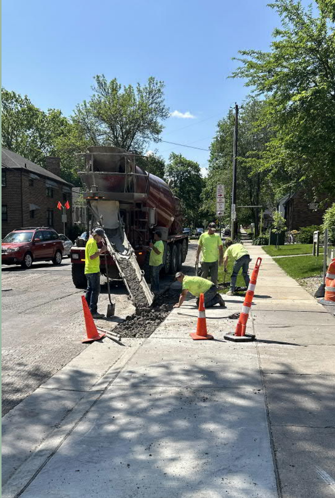
Driveway and Sidewalk Installation
