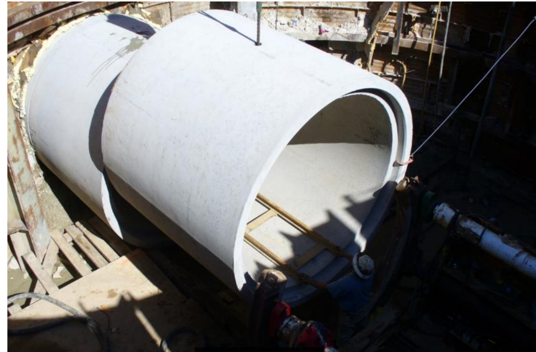
96" pipe tunneling on University Ave, Madison, WI (2013)
