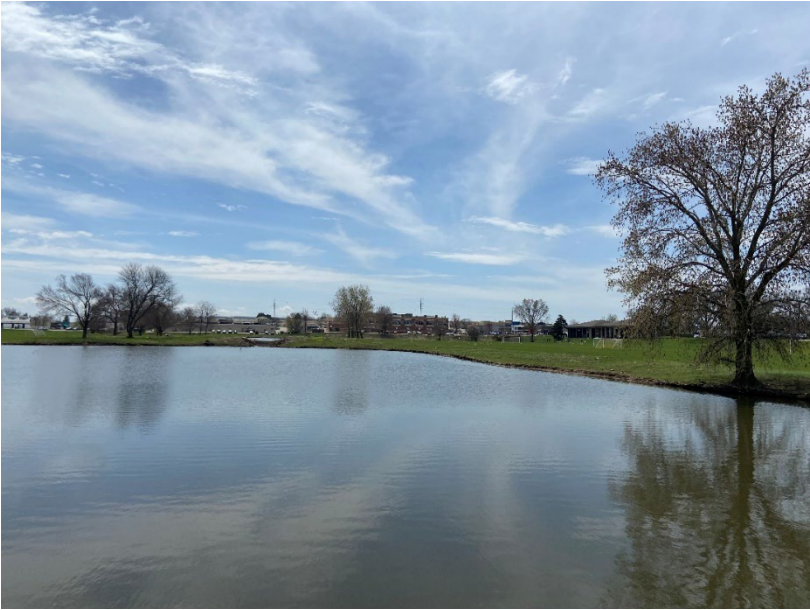
Looking From Outlet Structure on Mineral Pt. Road North
