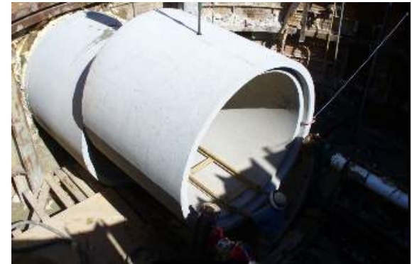
Above: 96" pipe on University Ave (2013)
