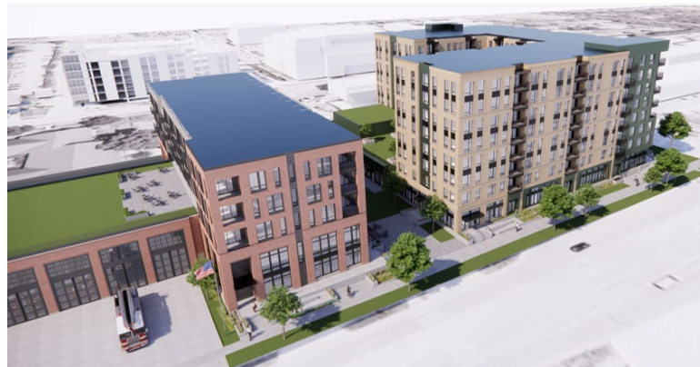
Exterior view, Badger Rd Aerial, Source:
